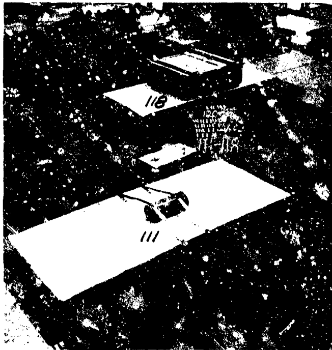
Fig. 323 - YOG 83 - Method of securing Items 111 and 116.
