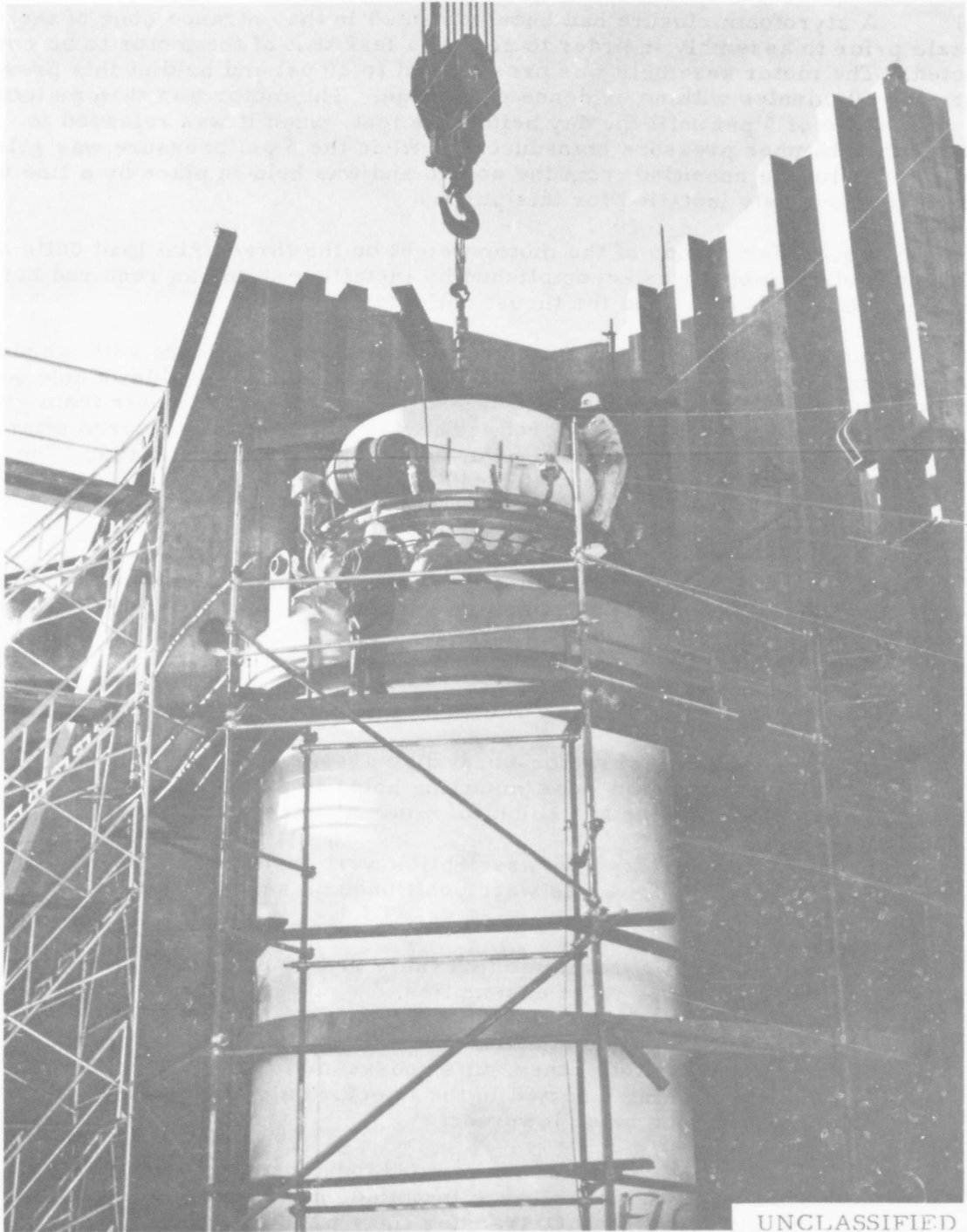
Figure 7 Motor 156-6 Nozzle Installation
