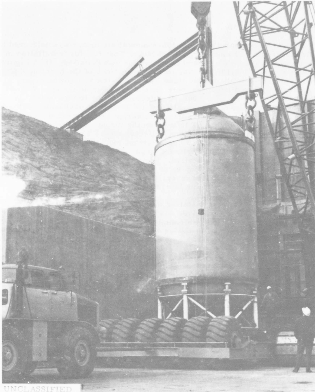
Figure 6 Motor 156-6 Installation in Thrust Stand
