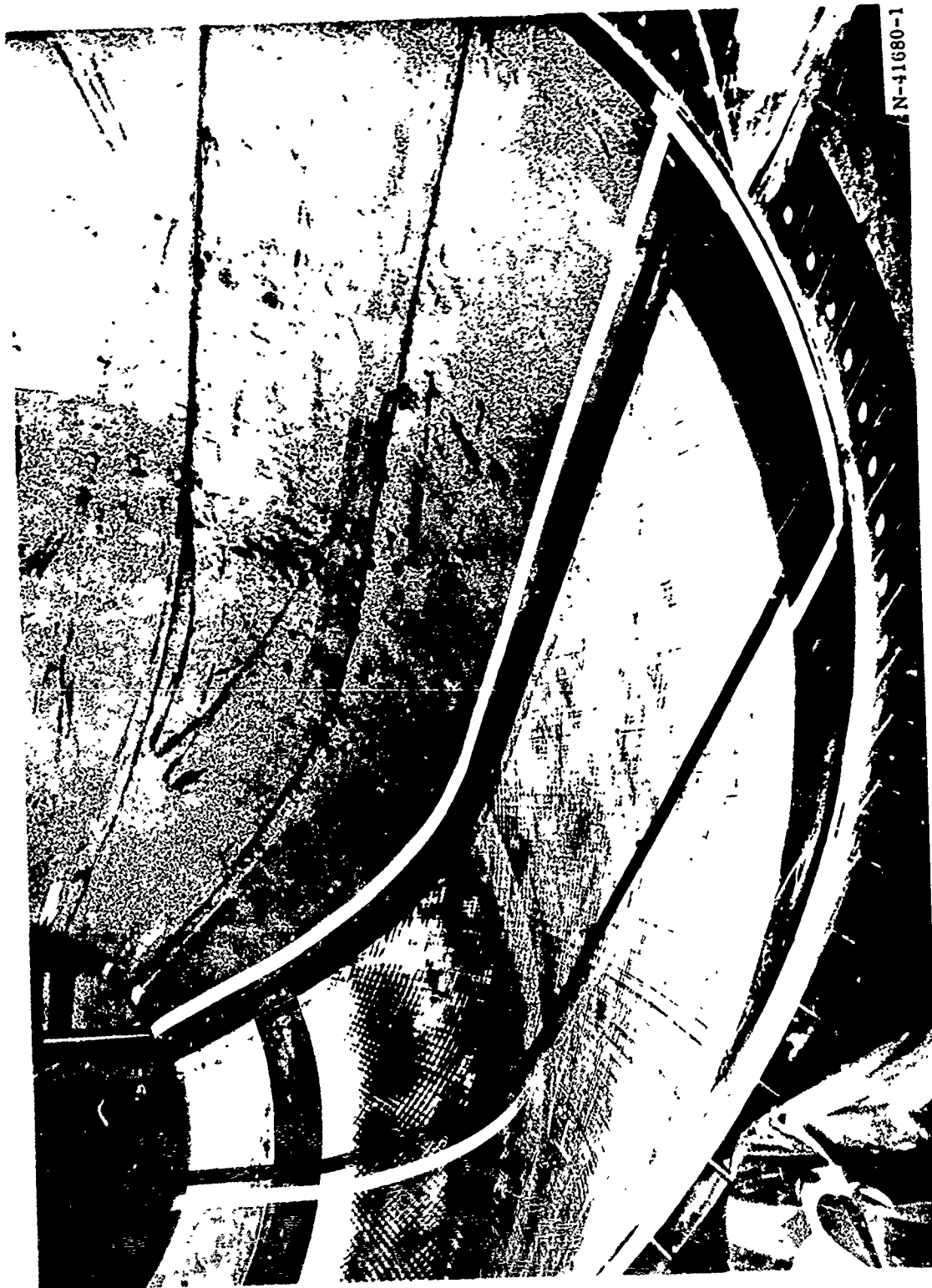
Figure 8. Replacement Bladder Partially Installed
