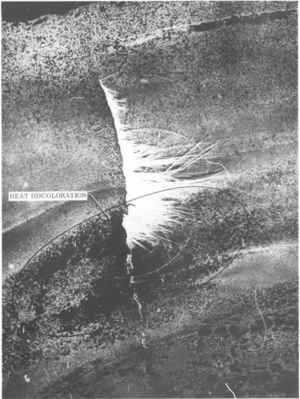
Figure 3. Area of Heat Discoloration
