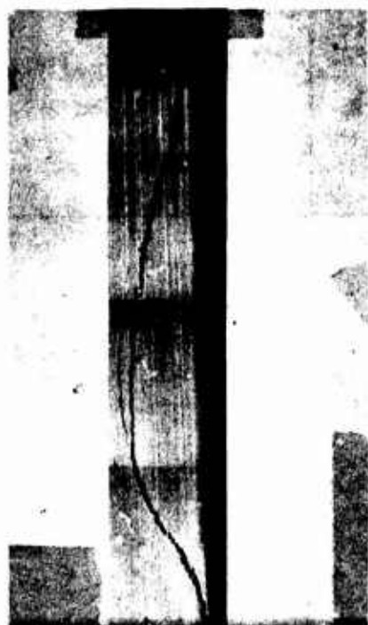
C Macro Crack found on inside surface
