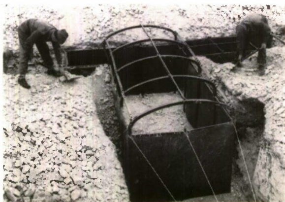
FIG. 9. Command Post Shelter.
