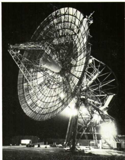
The 85 ft. parabolic antenna at the Deep Space Instrumentation Facility No. 41.
