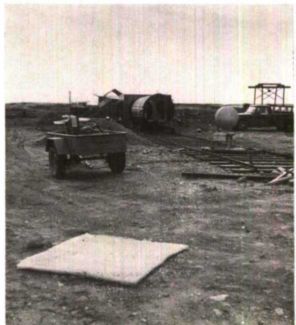
FIG. 9. Overall scene after fracture of the window.
