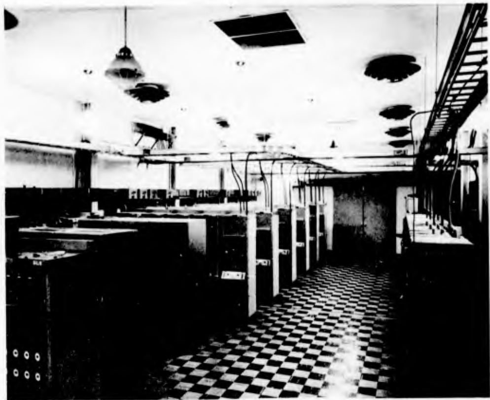
Fig. 1-4 Equipment room (looking south)
