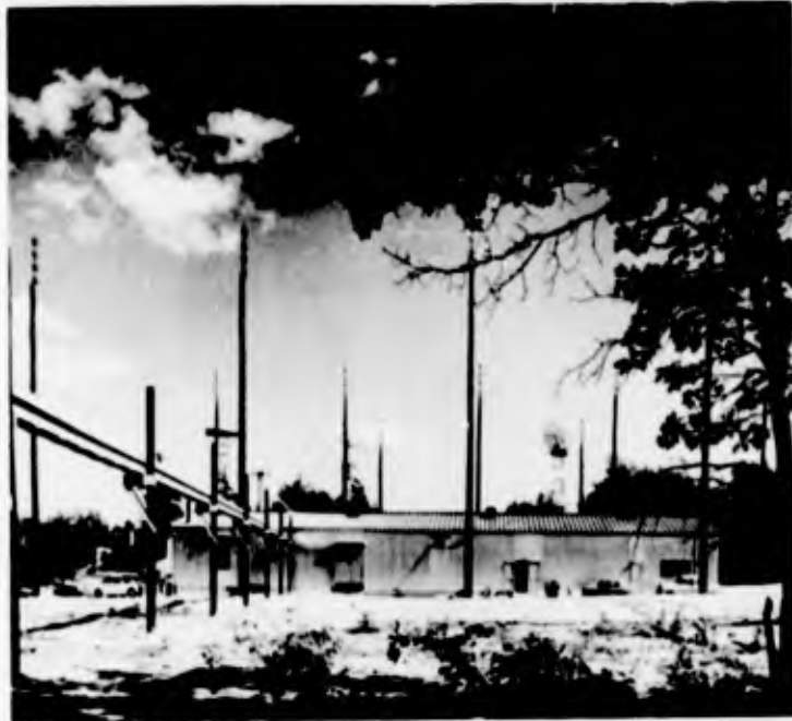
Operations building and antenna farm
