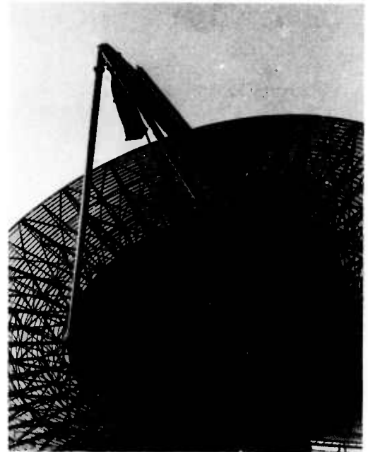
Fig. 9. Antenna, showing UHF waveguide run down to the rear of the dish and the heliax cable which carries the orthogonal polarization received signal.
