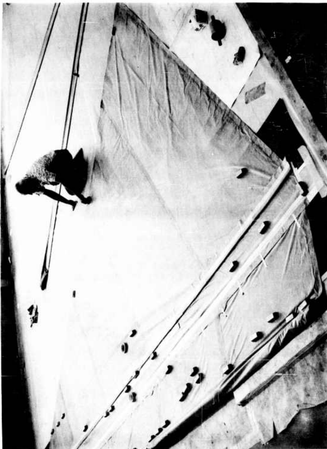
Figure 33 Membrane Assembly Complete
