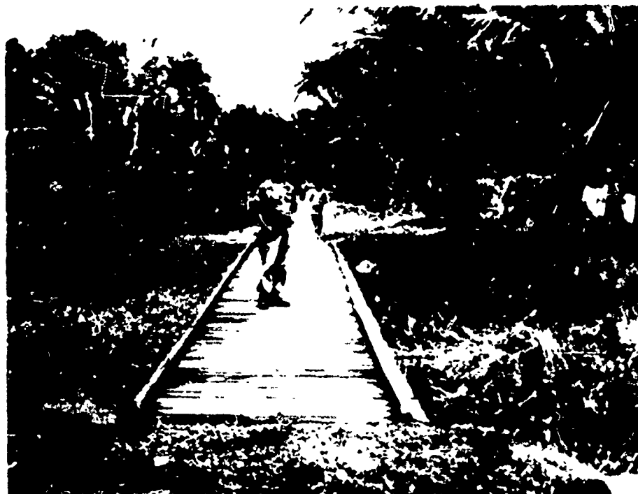
MAAG-3-11. Bridge viewed from the end. This bridge links 2 strategic hamlets. Lumber is not stocked in convenient sizes and lengths and must be ordered to size well in advance of requirements. Order-and-shipping times of 30 days are not uncommon in remote areas, where either timber source or milling facilities are not available.
