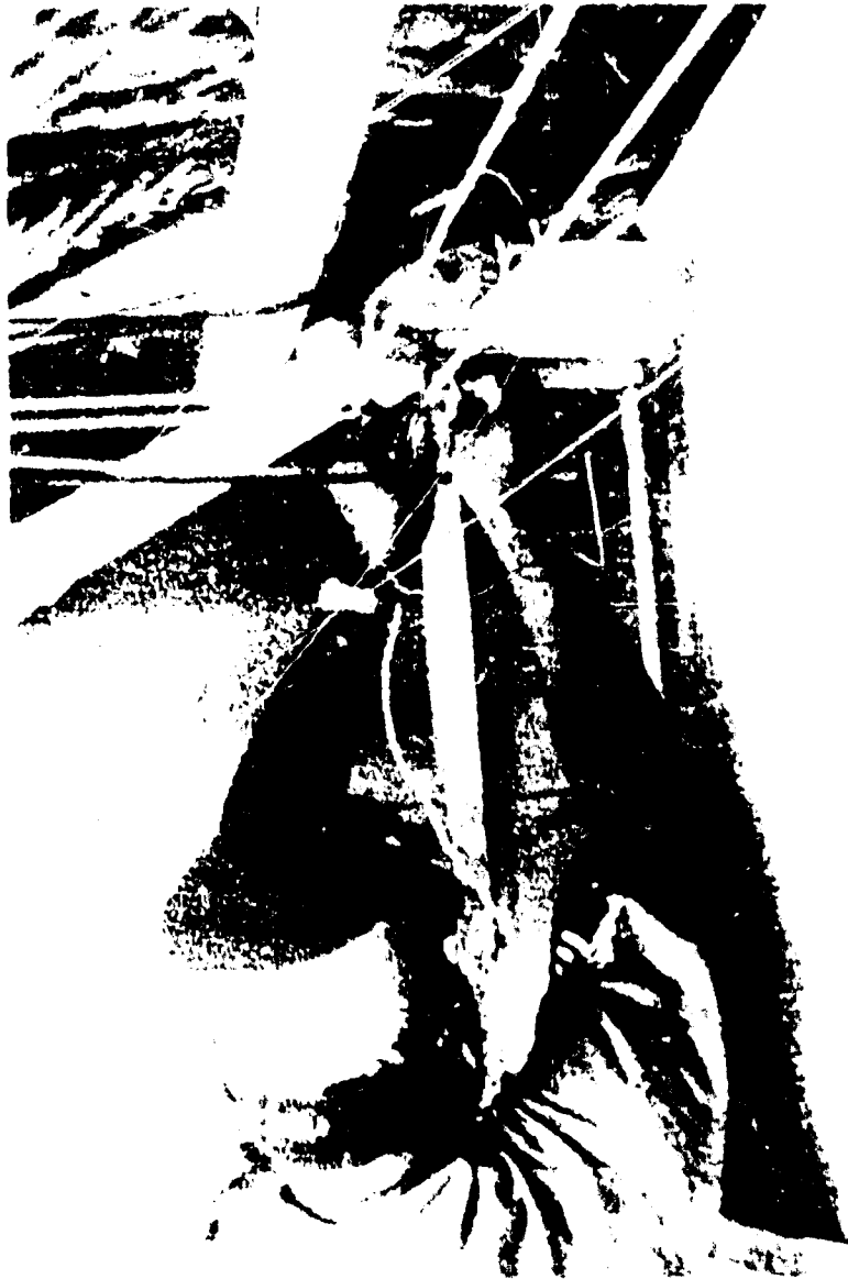
SF-2-14. A member of one of the two special forces ECAD advisory teams connects a new electrical line with an existing main line. Tie-in is being made to electric distribution system installed by a Vietnamese contractor. Note coil, to right of bamboo purlin, carefully wound to prevent having to cut and throw away a short section of excess wire.
