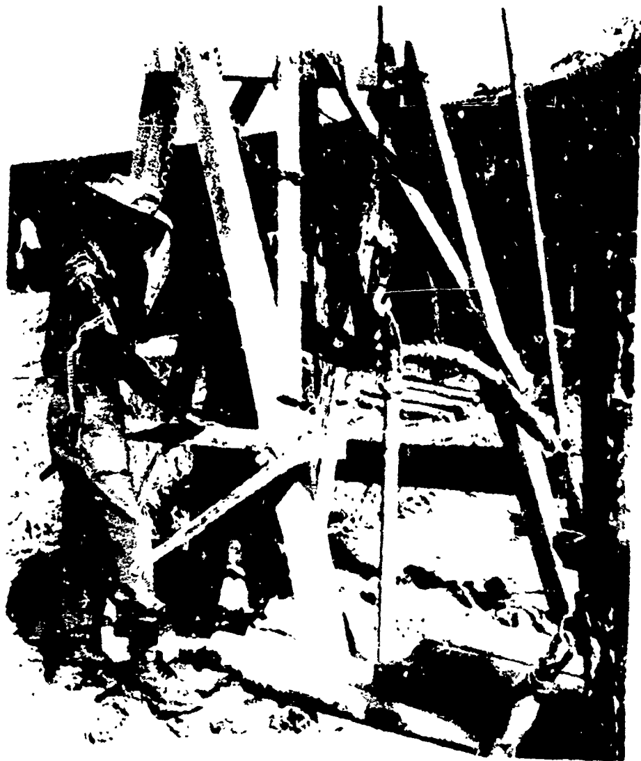
MAAG 2A-2. Sergeant Hicks supervising drilling operations. Four layers of different type clay were encountered in 220 foot depth.
