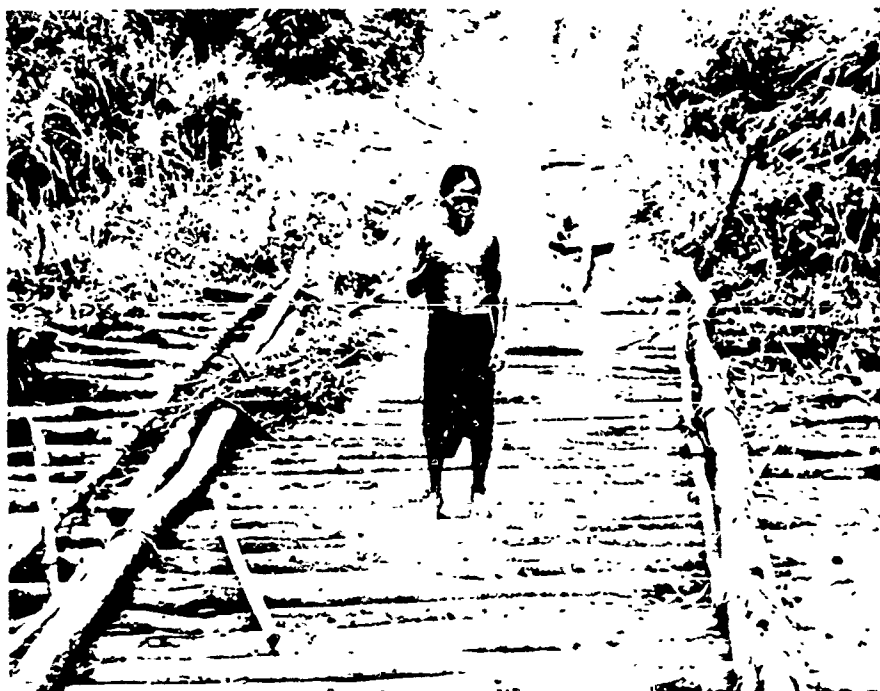
SF-1-2. Tactical bridge, 4 meters long, single span, class 20. Construction is of local material hewn from the adjacent jungle. This structure is used in support of clear and hold operations and is located approximately 7 kilometers west of POLIE KRONG. Old Montagnard woman tossed away a native cheroot in favor of an American cigarette offered by photographer. Debris on deck indicates mountain stream had overflowed its banks, with no damage to the bridge. Twelve-inch log stringers are placed on approximately 20-inch centers.
