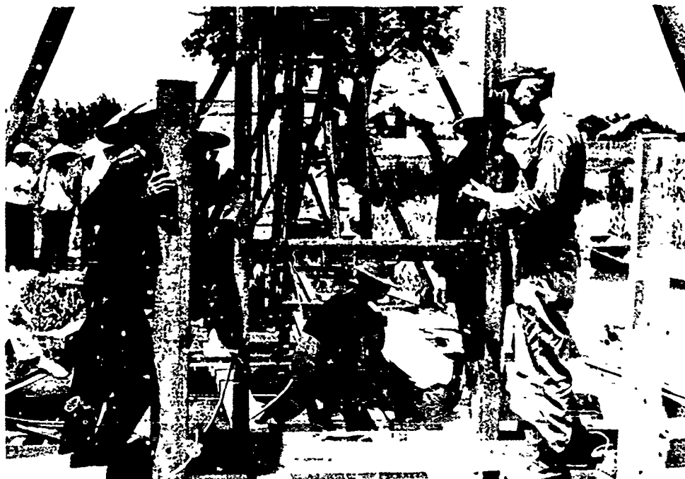
MAAG 2-1. Sergeant Mintz supervises local civil works personnel in erection of steel tripod on temporary platform at bailey bridge site.
