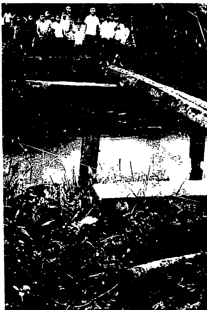
MAAG-3-6. Bridge site before construction of new bridge. Palm logs across bents provided for foot traffic. Concrete and timber bents from previous bridges can also be seen.
