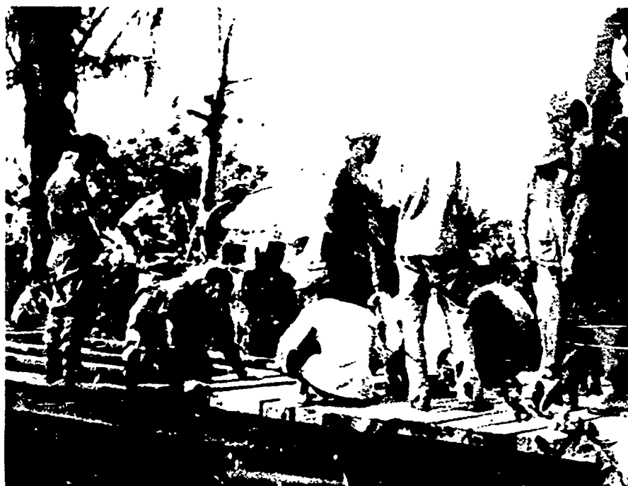
MAAG-3-7. Advisory team sergeant giving on-the-job training to unskilled hamlet civilians. Here Sergeant Vennes is showing workers how to space decking timbers. In some cases, unskilled workers had to be shown how to use a saw and hammer; in others, workers had some previous knowledge of the use of hand tools.
