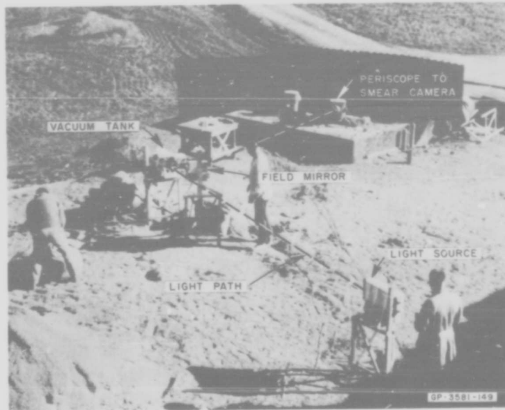
FIG. 19 ARRANGEMENT OF APPARATUS AT SMEAR CAMERA SITE FOR SHOT 9155 (U)
