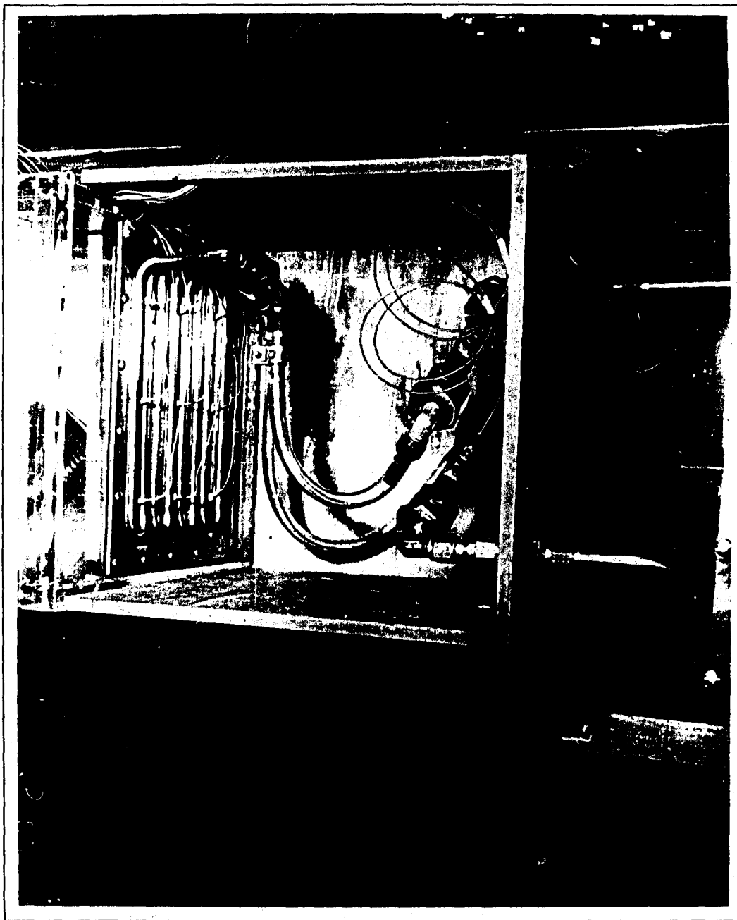
Figure 30. Connections from Plate to Flow Circuit
