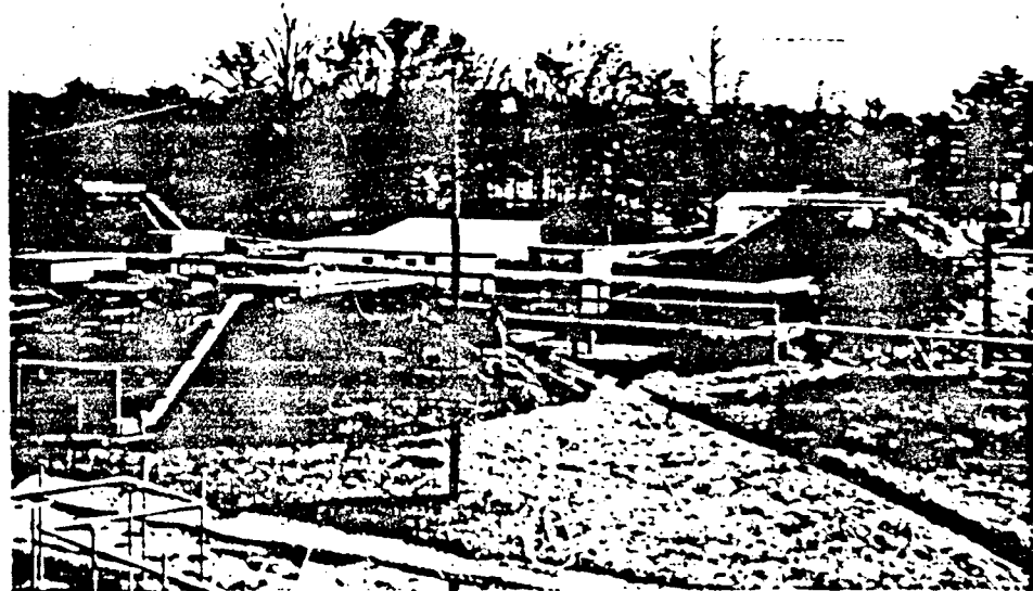
REMOTELY OPERATED MIXING AND PRESS BUILDING PROTECTED BY EARTH MOUNDS. NOTE: VENT TYPE ROOF-TUNNEL ENTRANCES ARE PROTECTED BY HEAVY SPECIALLY DESIGNED DOORS.
