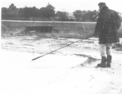
f. Lighted-torch proofing of vapor blanket
