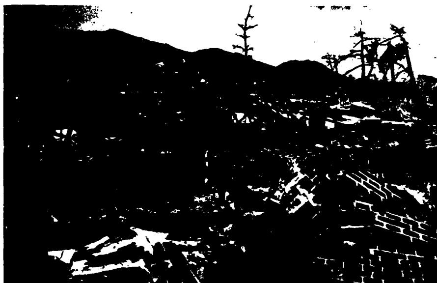
Building 84. Looking north along axis of building, showing complete collapse of walls and trusses by blast.
