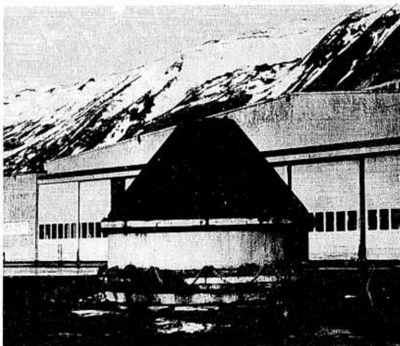
Figure 17A. Mooring buoy weighing over 10 tons now rests on the Station taxiway. Third tsunami wave cresting at 24 ft. above old MLLW drove this buoy inshore.
