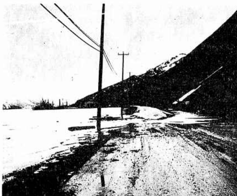
Figure 10. Kodiak Island subsidence of 5-1/2 feet allows high tide to wash over road to NRS(R) Holiday Beach. Cargo Pier in background.
