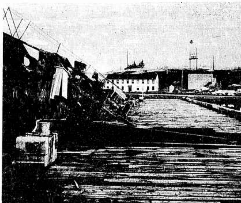
Figure 9. Moored barge under tsunami action pulled decking and bollard loose from marginal pier.
