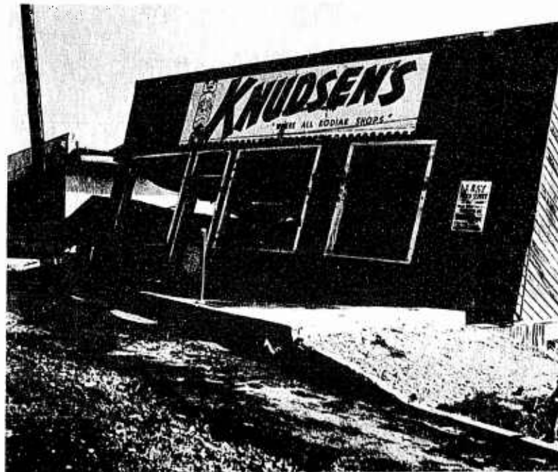
Figure 34. Haberdashery was washed right off its foundation and rested with its rear portion in the harbor.
