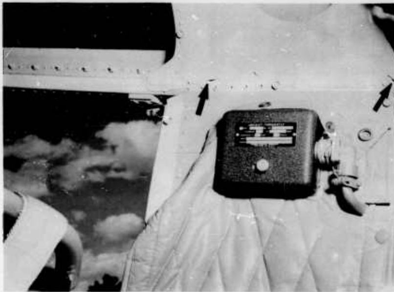
Figure 15. The arrows depicts the failures at the top of the right vertical side support.
