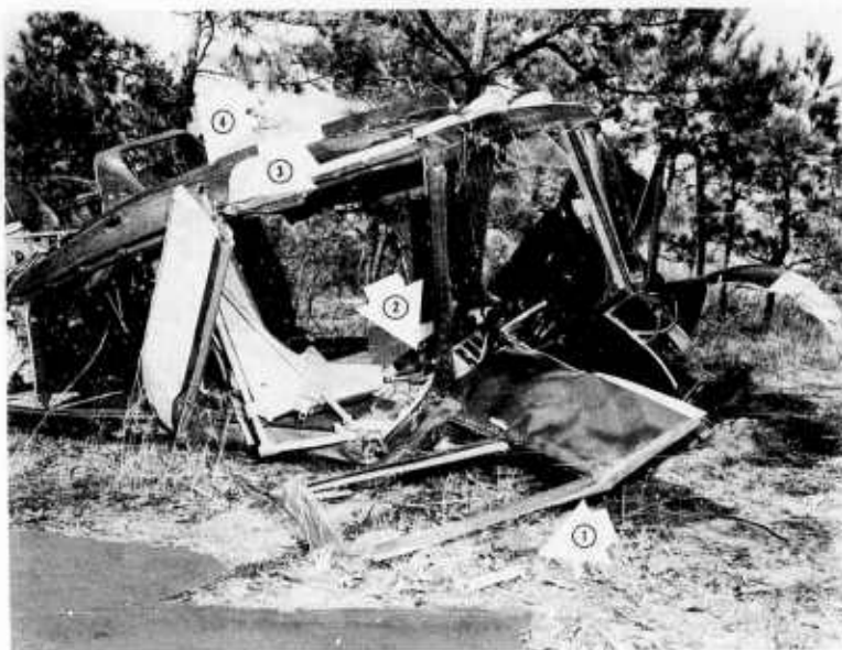
Figure 20. The collapse of the aft bulkhead allowed the roof structure to impinge into the occupiable area in Accident "B".
