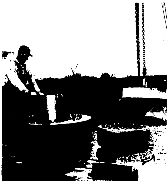
A cylindrical Monel blank (actually two welded Monel cylinders telescoped within one another) is placed in a heavy laminated steel die. The assembly is partially filled with water and a stick of dynamite suspended at water level. The heavy block shown suspended at right is placed over the die.
