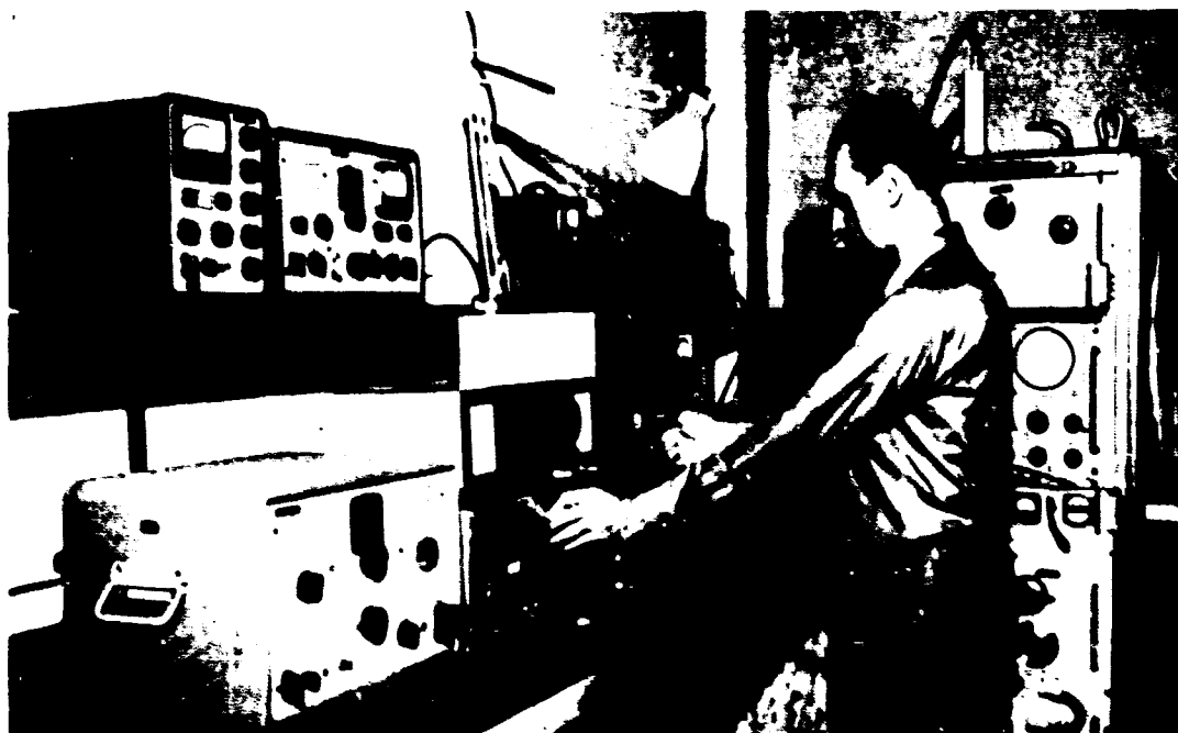
Fig. 7 CALIBRATION OF RECEIVER IN INSTRUMENTATION LABORATORY
