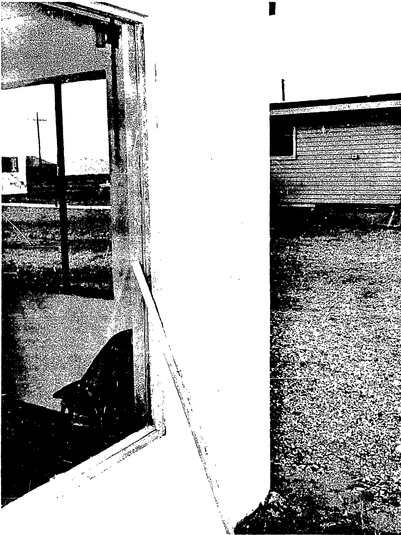
Fig. IX-6 Molding on 5' x 10' x 1/4" Window Popped off During a 38 psf Boom. Note that Only One Nail Held the Molding and that the Window Did Not Break. None of 12 Windows of this Size Broke on this Critical Vector Boom.
