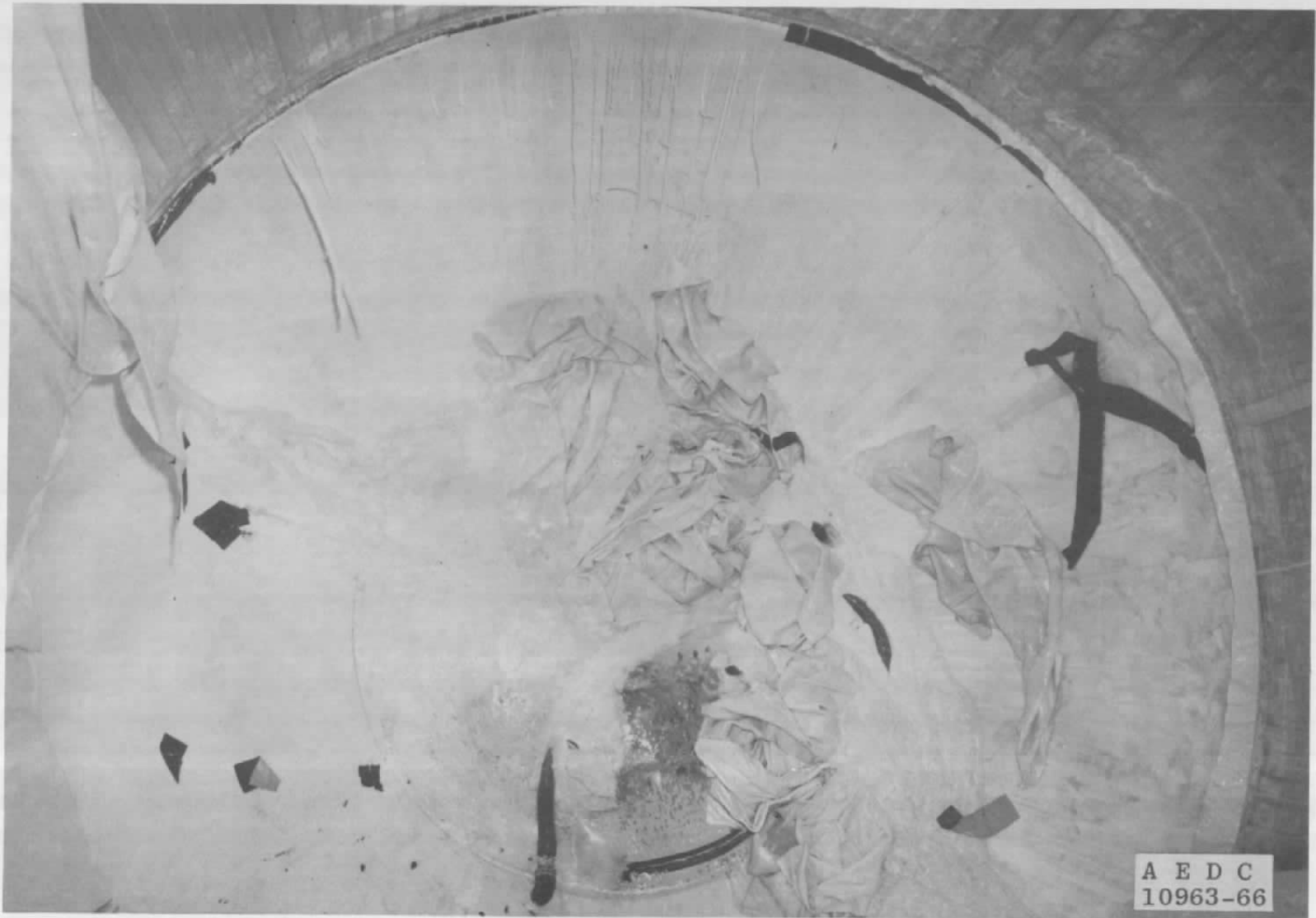
Fig. 17 Inside of Lower Bulkhead after Shelter Rigidization
