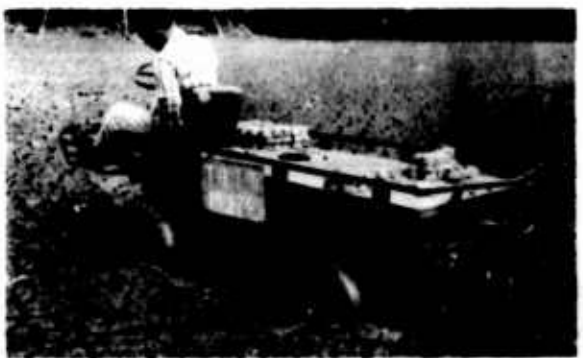
Fig. 27. M274 with 7.50-10 tires. Immobilized on 1st pass.
