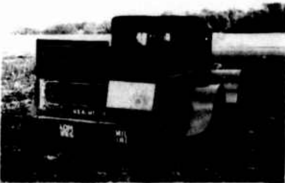
Fig. 31. M37 with 9.00-16 tires. Immobilized on 1st pass.
