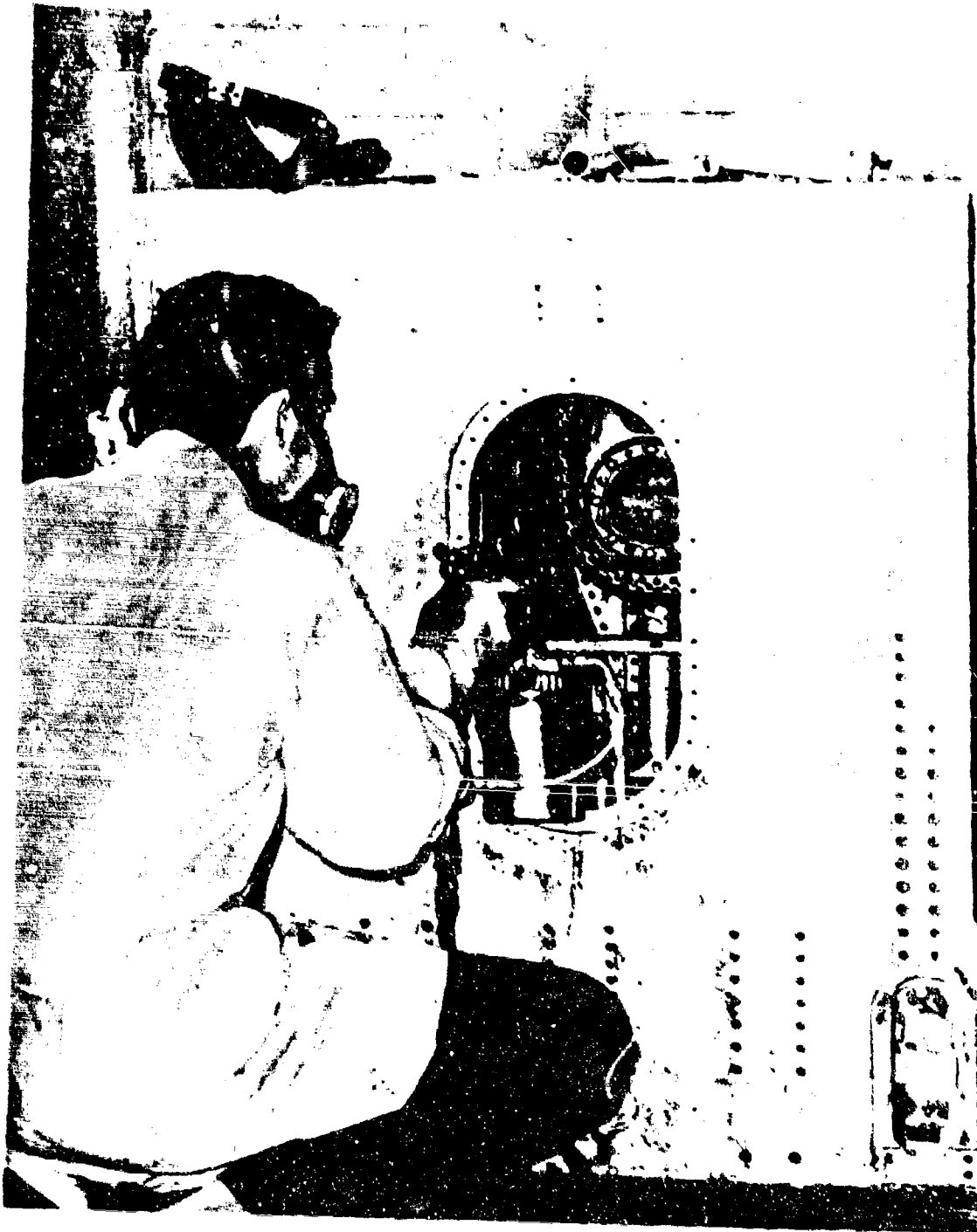
Spray application of coating formula 2414-501.4 to integral fuel tanks.
