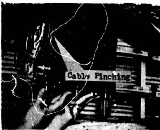
FIGURE 3-8. Cramped Cabling Around High Voltage Power Supply
