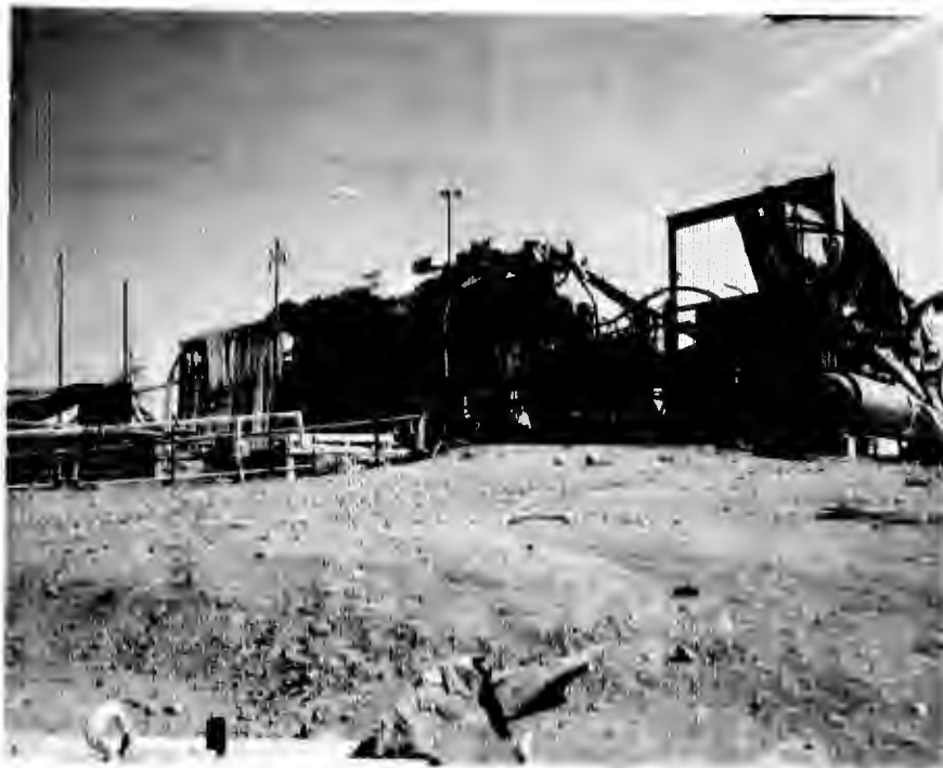
Figure 159. NFL-B4A Facility Damage (viewed from block house side) (U)
