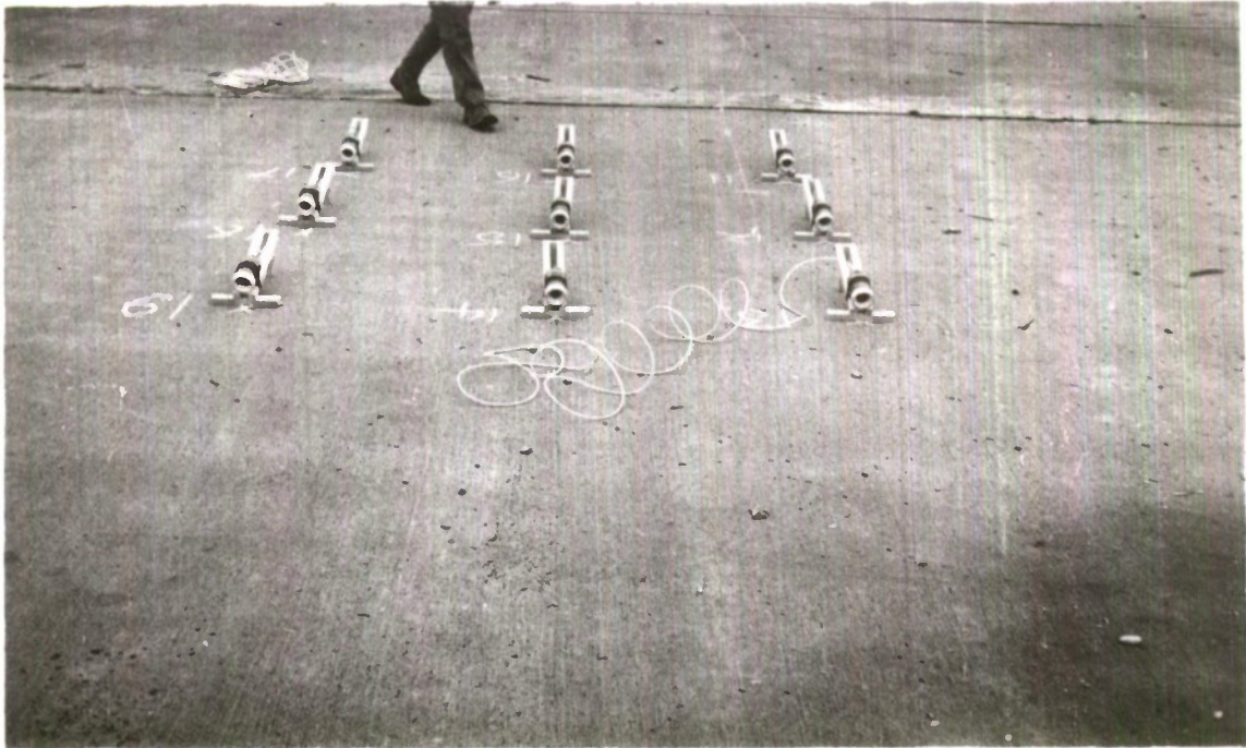
FIG. 2(a) SHAPED CHARGES SET FOR FIRING AT WEST FREUGH
