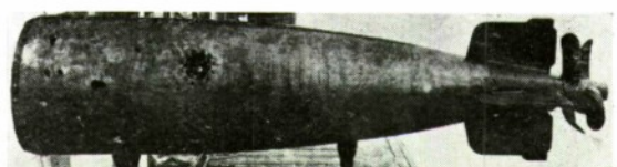
FIG. 20. Tail of 19.7in. German Torpedo (1917). Note curved propellers.
