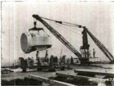
The 3D Radar Aerial being installed at ASRE in 1953 in the new "3D Radar Building". This was the first experimental radar fitted at ASRE, Portsmouth.
