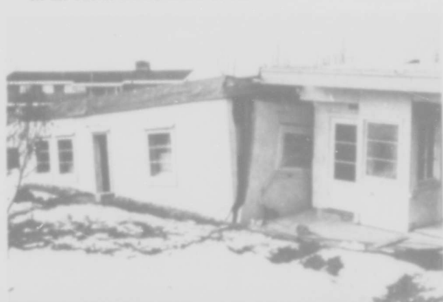
Figure 22.--Poor corner reinforcing is evident in this house with poured concrete walls damaged in an earth subsidence area.
