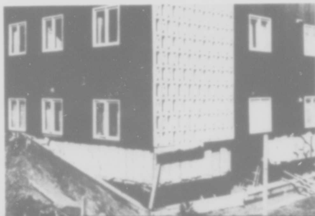
Figure 12.--The rigidity of the wood framed wall is clearly evident in this three-story apartment building.
