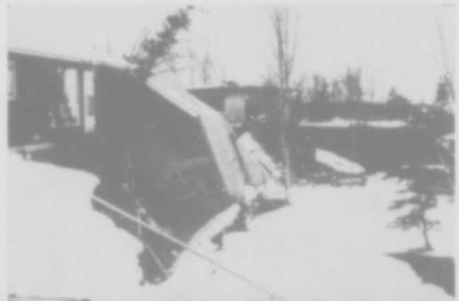
Figure 26.--Even though this wood frame house had dropped into an earth slide area, the roof remained rigid and essentially undamaged.
