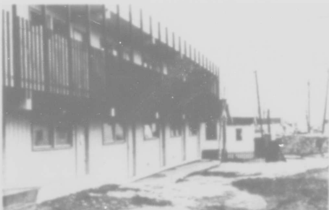
Figure 16.--Although this wood frame apartment building had dropped almost 6 feet, the plywood-faced panels helped to minimize damage. ZM 126 455
