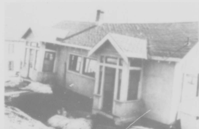
Figure 18.--Although the earth dropped under this house, the wood sheathing and stucco exterior provided a good shear wall. ZM 126 456
