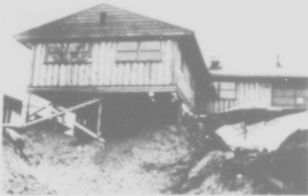
Figure 3.--Wood frame home in Turnagain bluff area. Earth subsidence destroyed a portion of the basement but caused little harm to house. Temporary bracing has been placed under the left portion.
