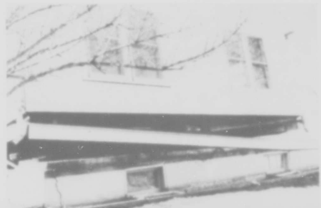
Figure 6.--Inadequate fastening of wall to floor system caused some floor damage. Little racking of the house was apparent though one end had fallen into an earth fault.
