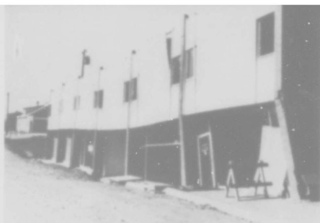
Figure 32.--The wall of the second floor offered some resistance to racking forces; not so the open first floor, which lacked enough reinforcement to resist lateral movement.
