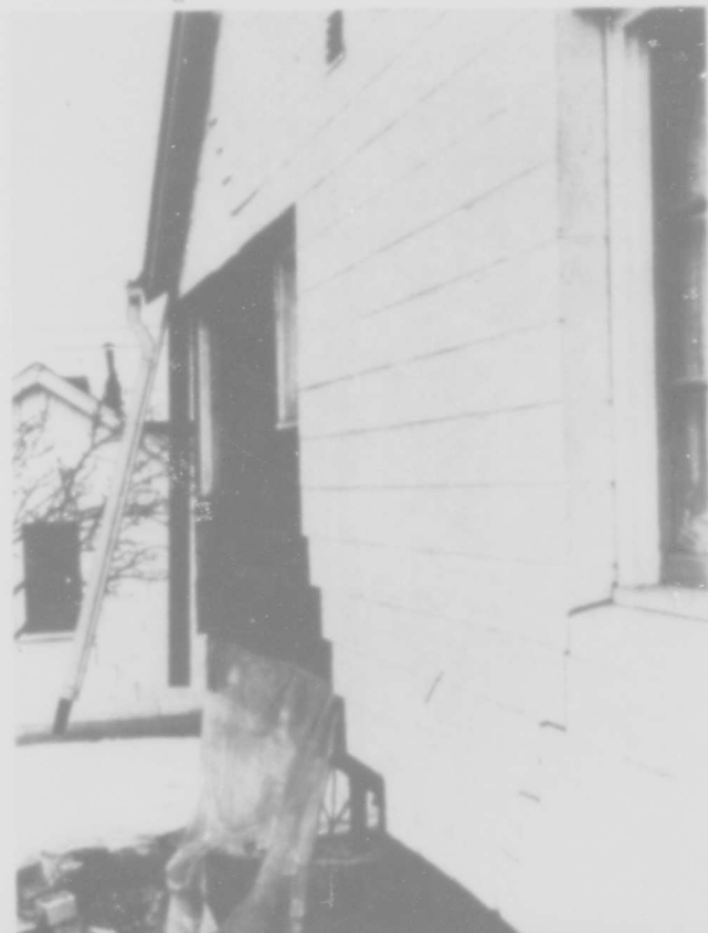
Figure 20.--The nonflexible facing of masonry failed but the more flexible wood wall framing remained undamaged.
