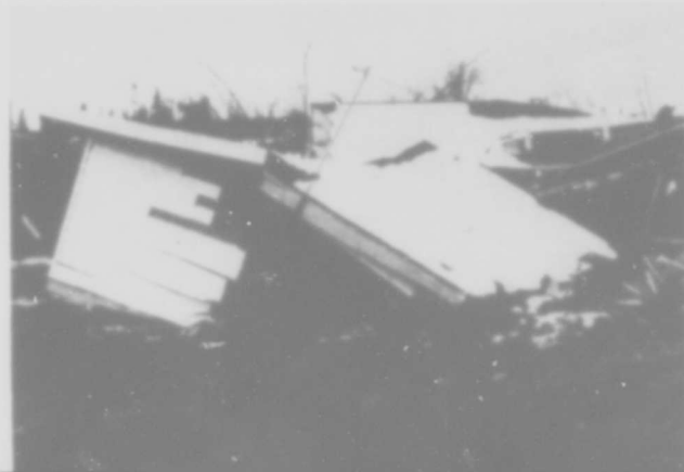
Figure 14.--The impact of the sudden earth subsidence was sufficient to cause shearing of the fiberboard sheathing.
