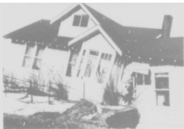
Figure 19.--The drop siding without use of sheathing did not provide enough rigidity to prevent damage to this house.
