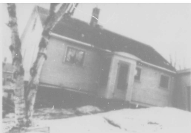
Figure 15.--Wood sheathing and siding over a wood framework, together with good nailing, provided strength and rigidity in this house.
