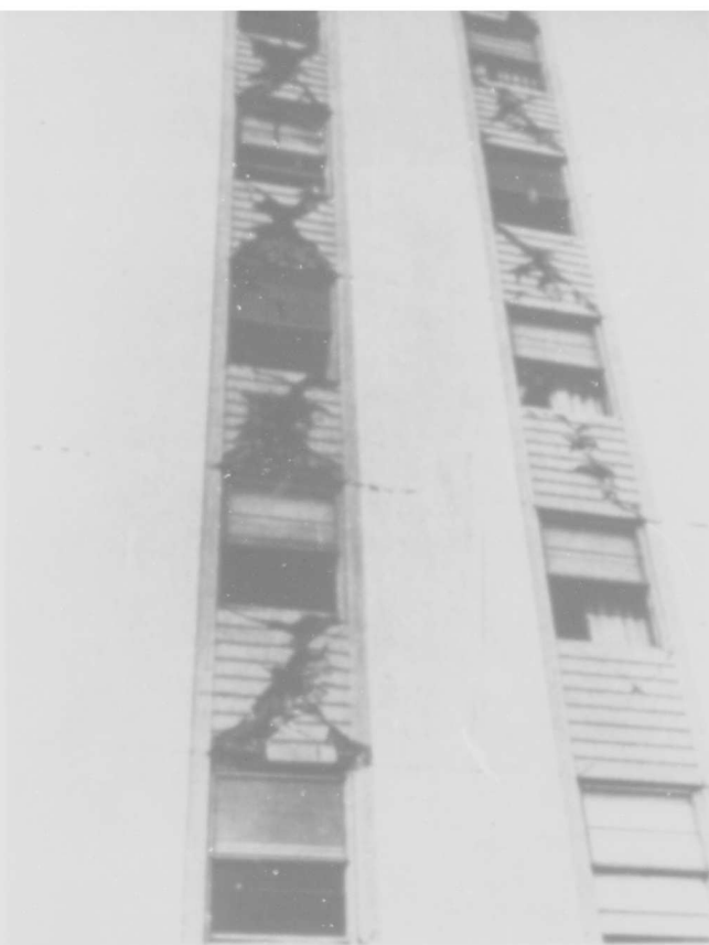
Figure 33.--The reinforced spandrel panels over the windows failed in shear. Shear failures at each floor line are also visible.
