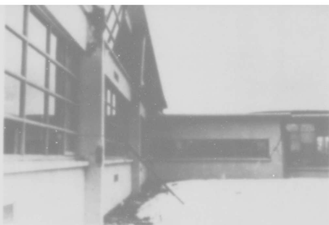
Figure 31.--The widely spaced columns of this school offered little resistance and failed at points of fixity at floors and roof line.
