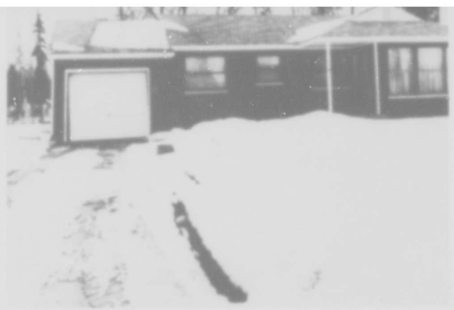
Figure 5.--Fissure in earth (center, foreground) caused slight movement of floor slab and twisting of garage door. This home is near the Turnagain housing area where severe earth slides occurred.
