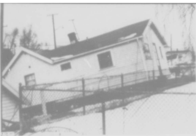
Figure 27.--Both roof and wall rigidity prevented major damage to this house.
