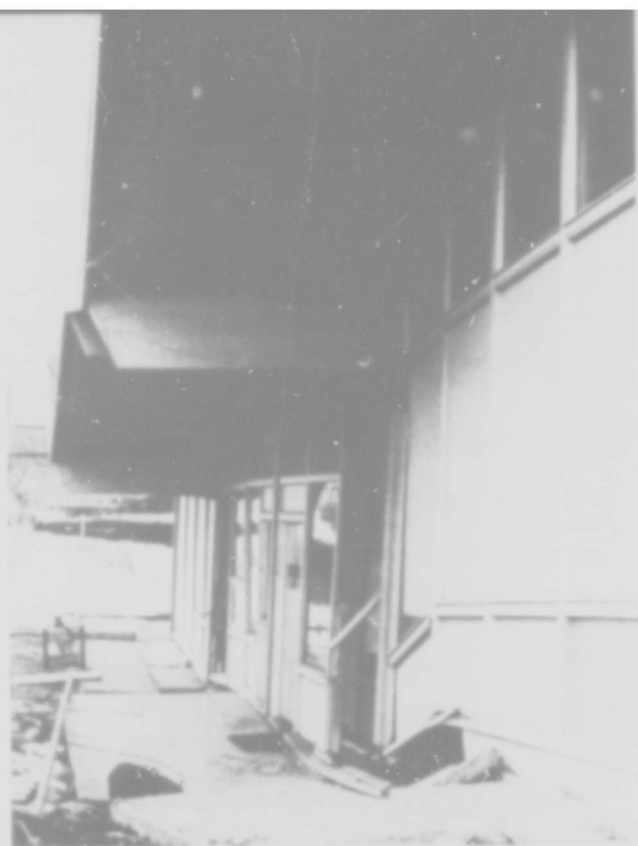
Figure 9.--This one-story office building constructed on a concrete slab was racked and badly damaged in an earth subsidence area, primarily because of slab failure. Wood roof decking and laminated beams are practically undamaged.
