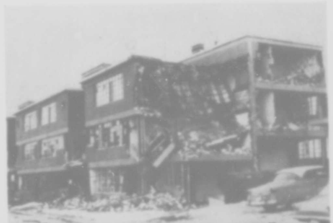
Figure 30.--Resistance to racking forces of the earthquake was lacking in this apartment building.
