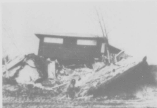
Figure 10.--Although this wood house had been exposed to earth slides as well as shocks from the earthquake, only moderate damage to the structural frame was apparent.
