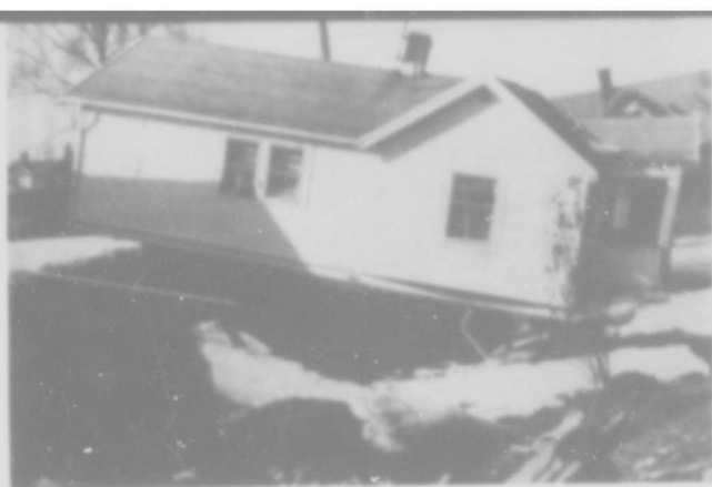
Figure 7.--Although the porch is somewhat awry, this small wood frame house was rigid enough to span the hole caused by earth subsidence.
