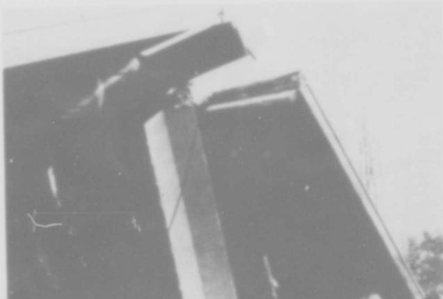
Figure 28.--Nail-laminated ridge beam separated, causing roof failure of this attached garage.
