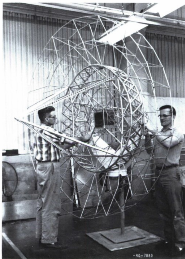
Fig. 4. 1/15 scale model of Haystack antenna.
