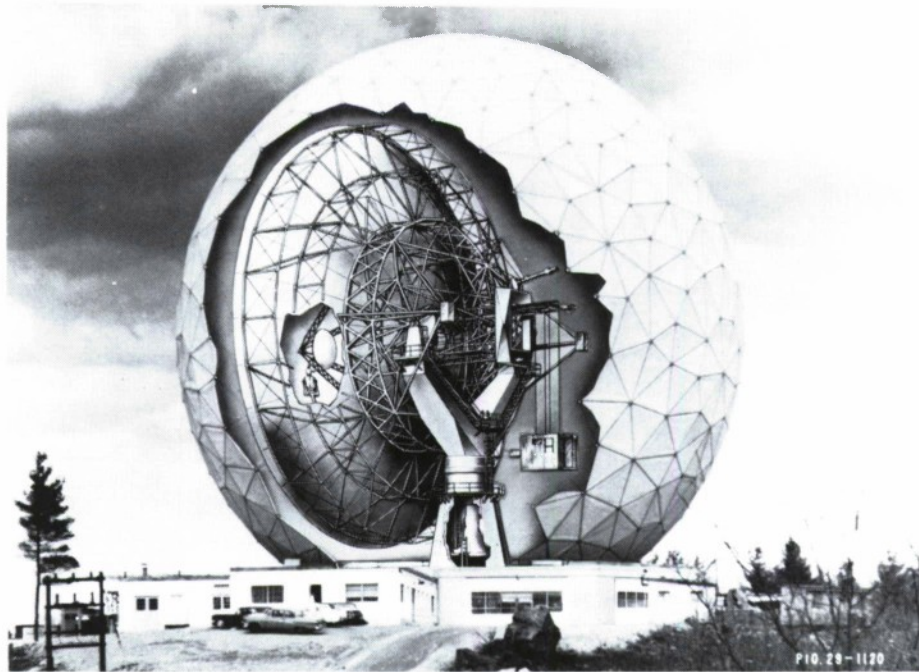
Fig. 16. Placement of antenna within radome.
