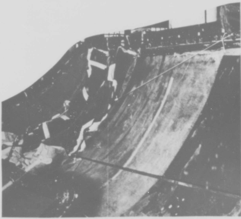
FIGURE 89 RESTRAINT OF 15^{\circ} PLUS DURING SPLICE FABRICATION
