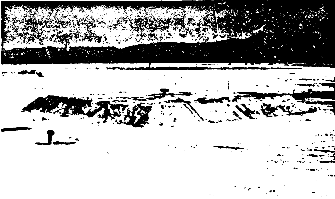
Figure 2.51 Earth-cover configuration of Structure 3.3c (preshot).
