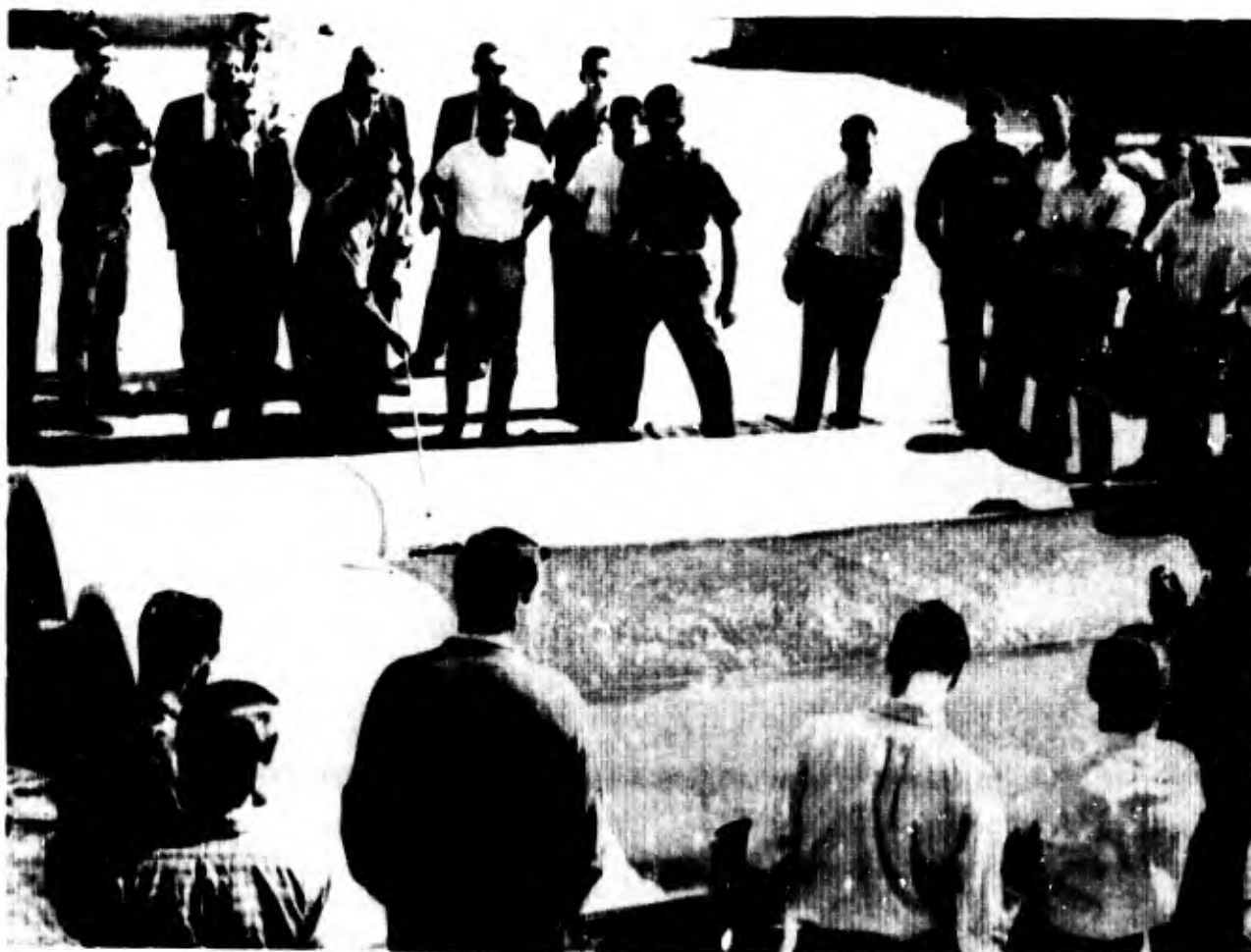
Waterproofing Assembled Units
