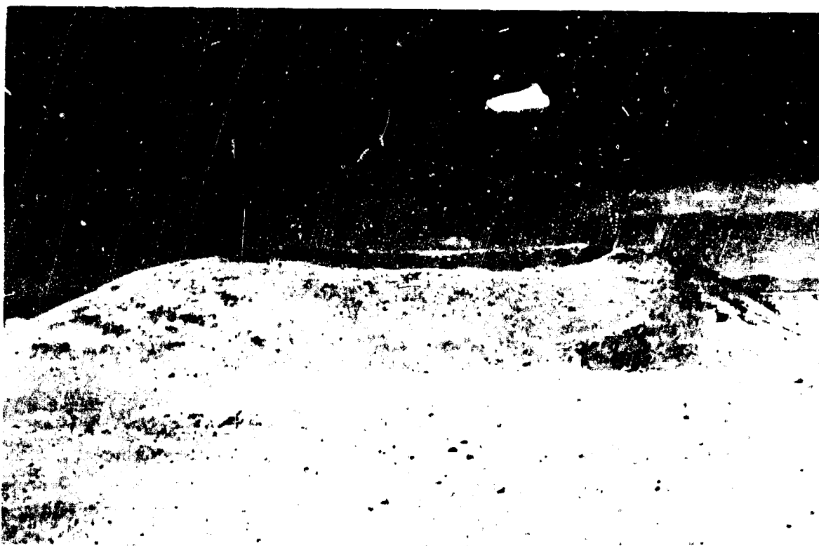
Figure 4.4 Earth berm, Building 3.6, after shot.
