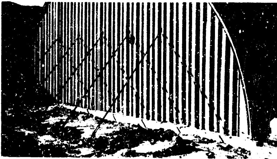
Figure 2.4 End-wall strengthening.
