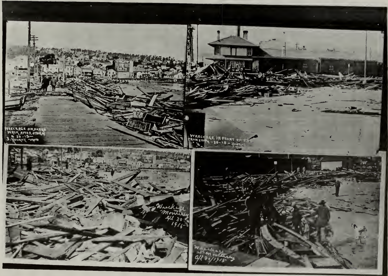
Fig. 8. Damage from the storm of 29 April 1915.
