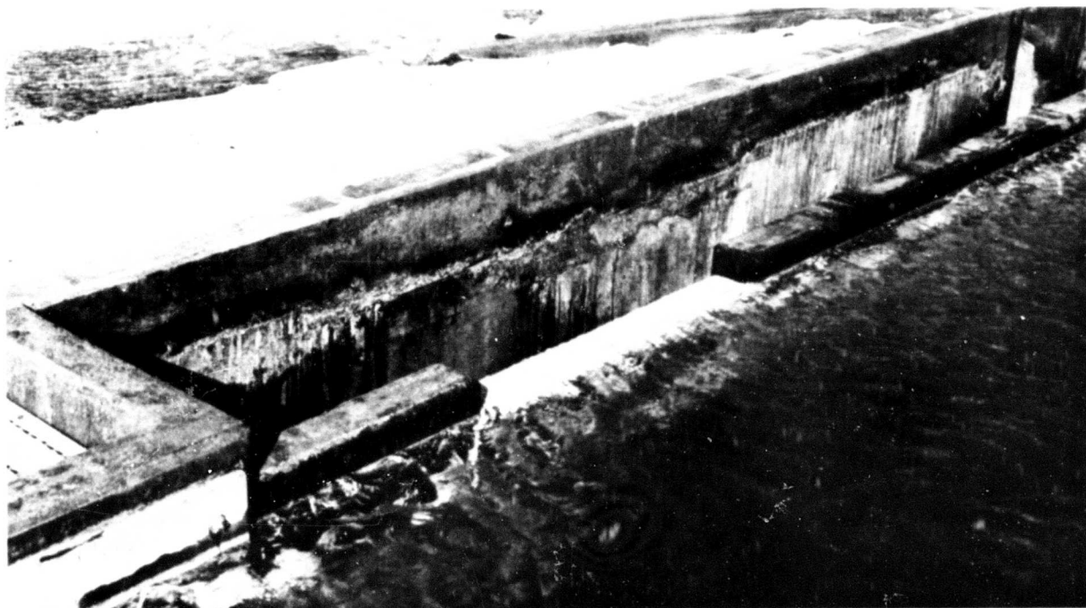
FIGURE 11. Closeup of Repaired Wall and Wier Section. Calcium Aluminate Bonded Refractory Concrete Used to Repair Top Section.
