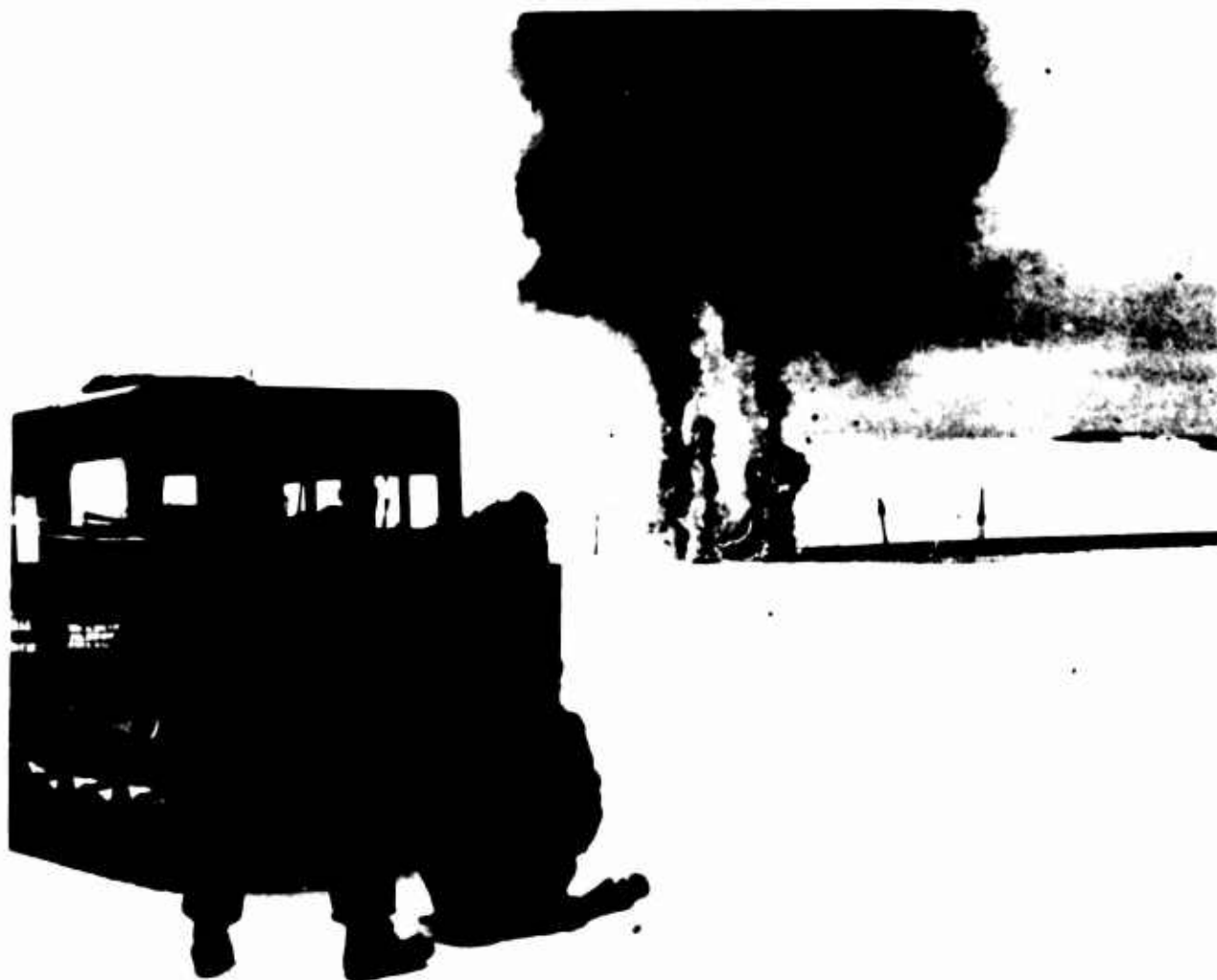
Figure 34. Blowing the snow bridge of a crevasse near the edge of the Greenland Ice Cap during trail operations.
