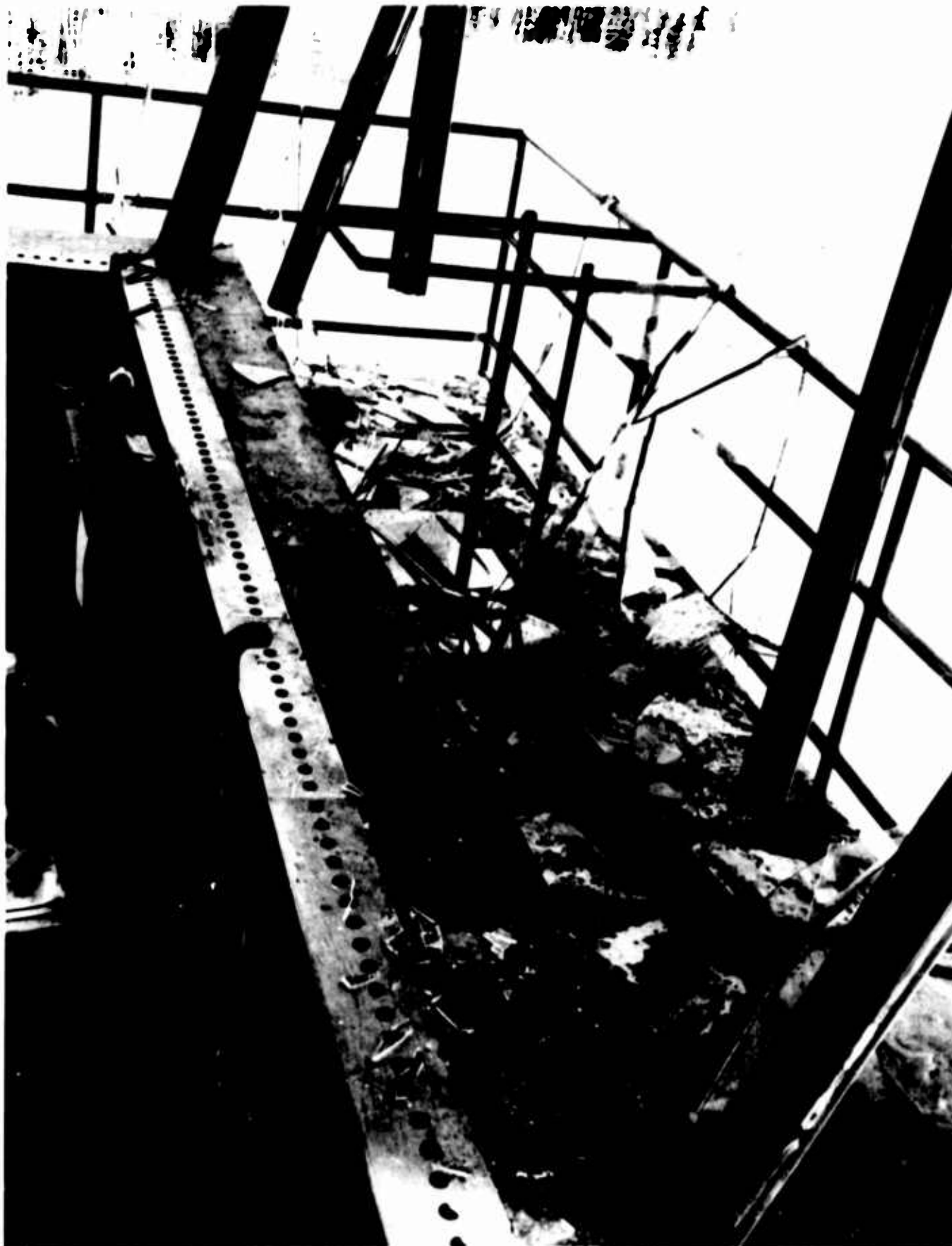
Figure 133. Elmendorf AFB Aircraft Control Tower (Severely damaged observation cupola)
