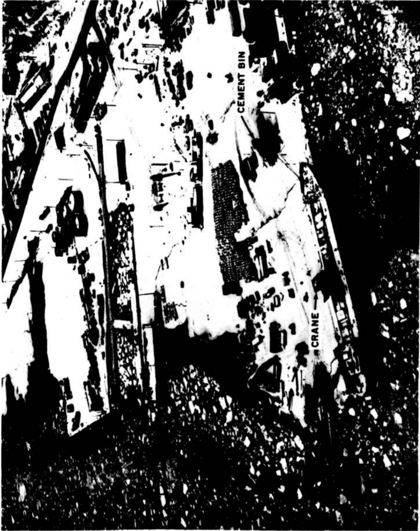
Figure 243. Alaska Aggregate Corporation Dock (Aerial view showing fallen crane and cement bin)
