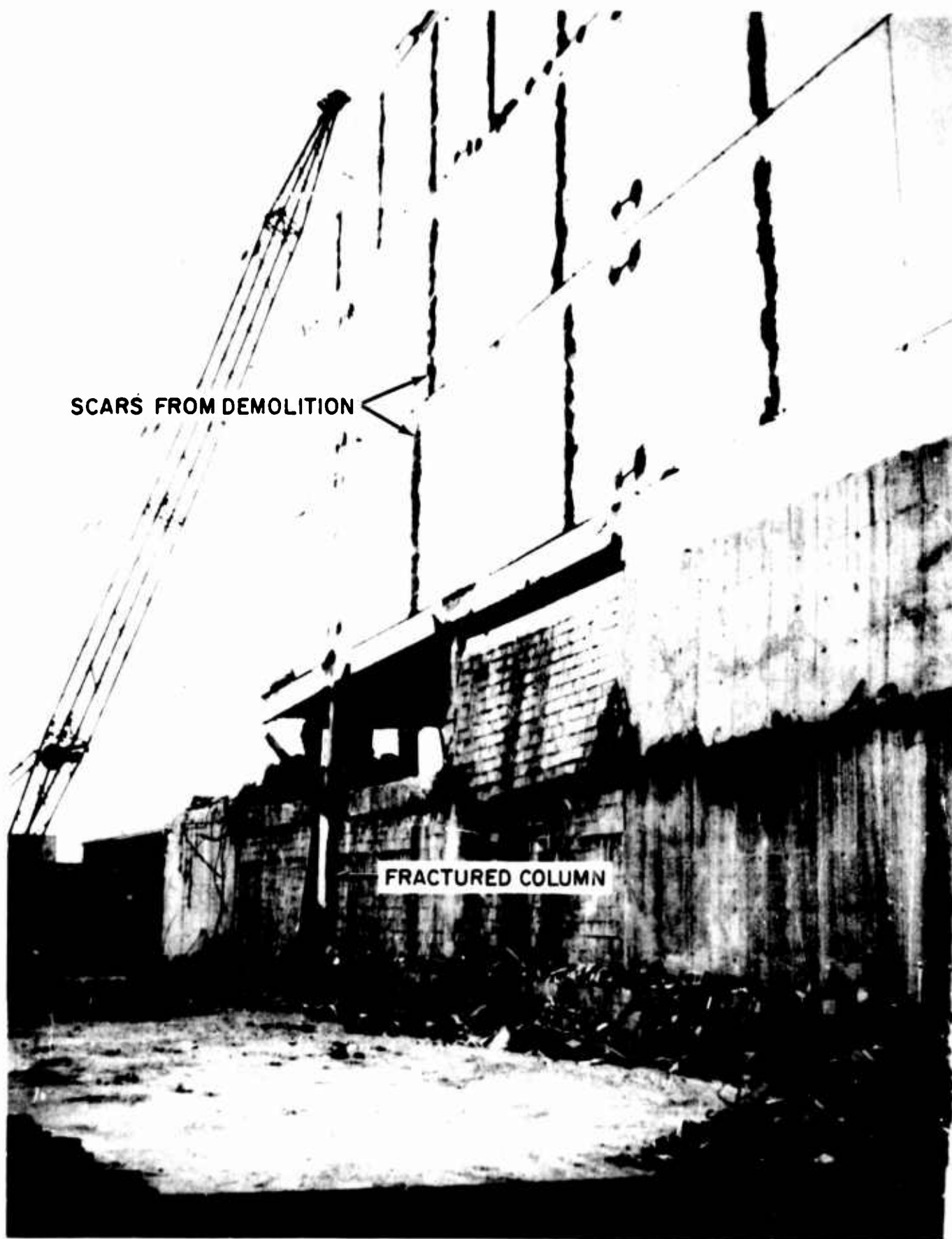
Figure 142. J. C. Penney Building (West side of the structure during demolition showing unseated shear panels and fractured column. Adjacent building has been razed to make room for demolition operations.)
