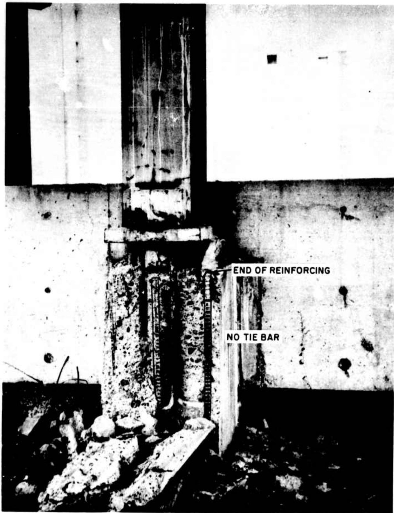
Figure 226. Alaska Brewery Company Structure (Severe damage to an exterior footing without horizontal ties)
