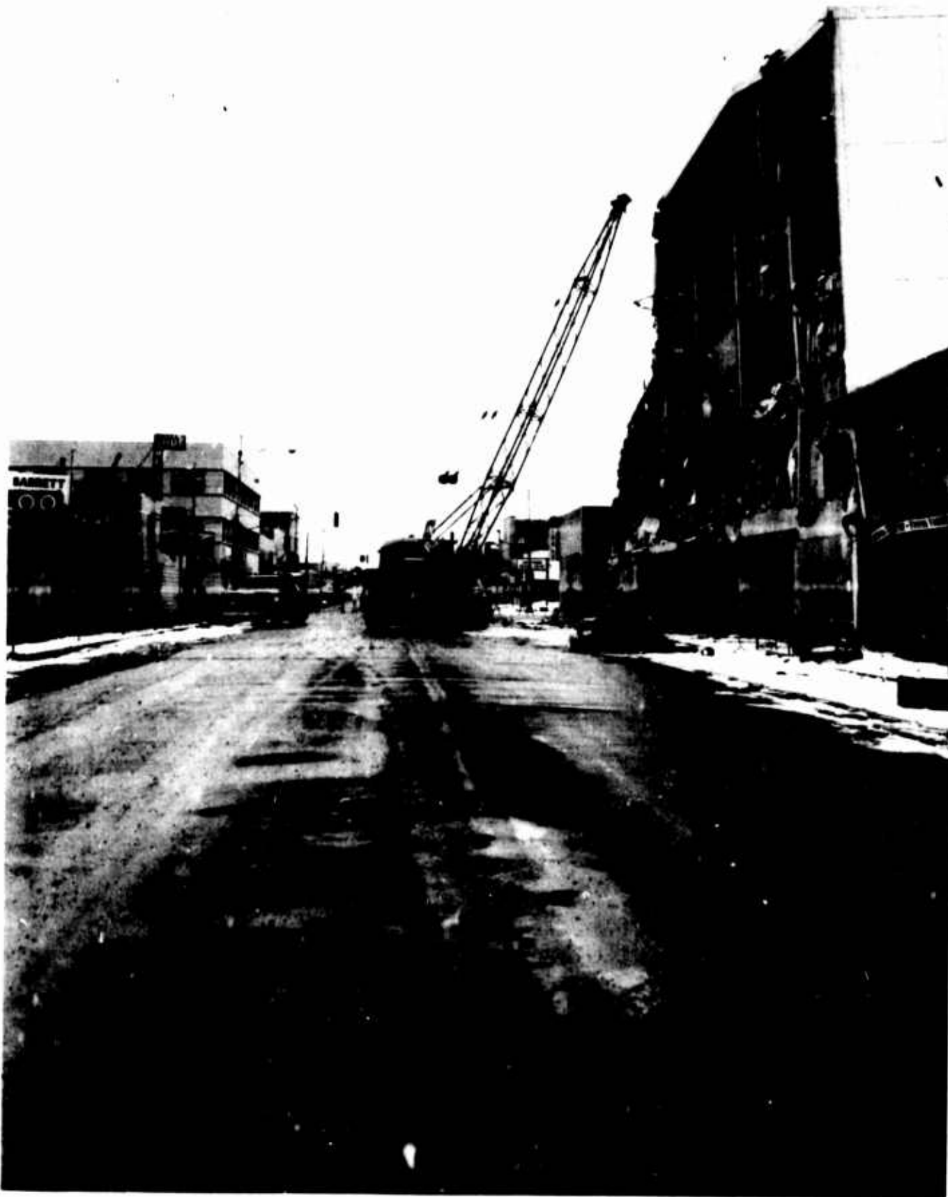
Figure 140. J. C. Penney Building (Damage to the northwest corner of the structure. Notice numerous floorslab failures.)
