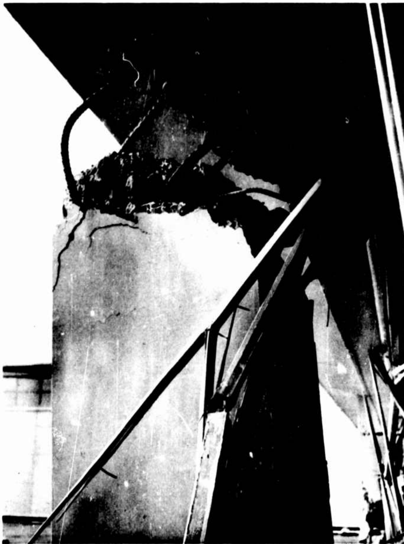
Figure 180. West Anchorage High School (Complete fracture of a second-story column in south wall of wing B. The reinforcing steel is bent but not broken.)
