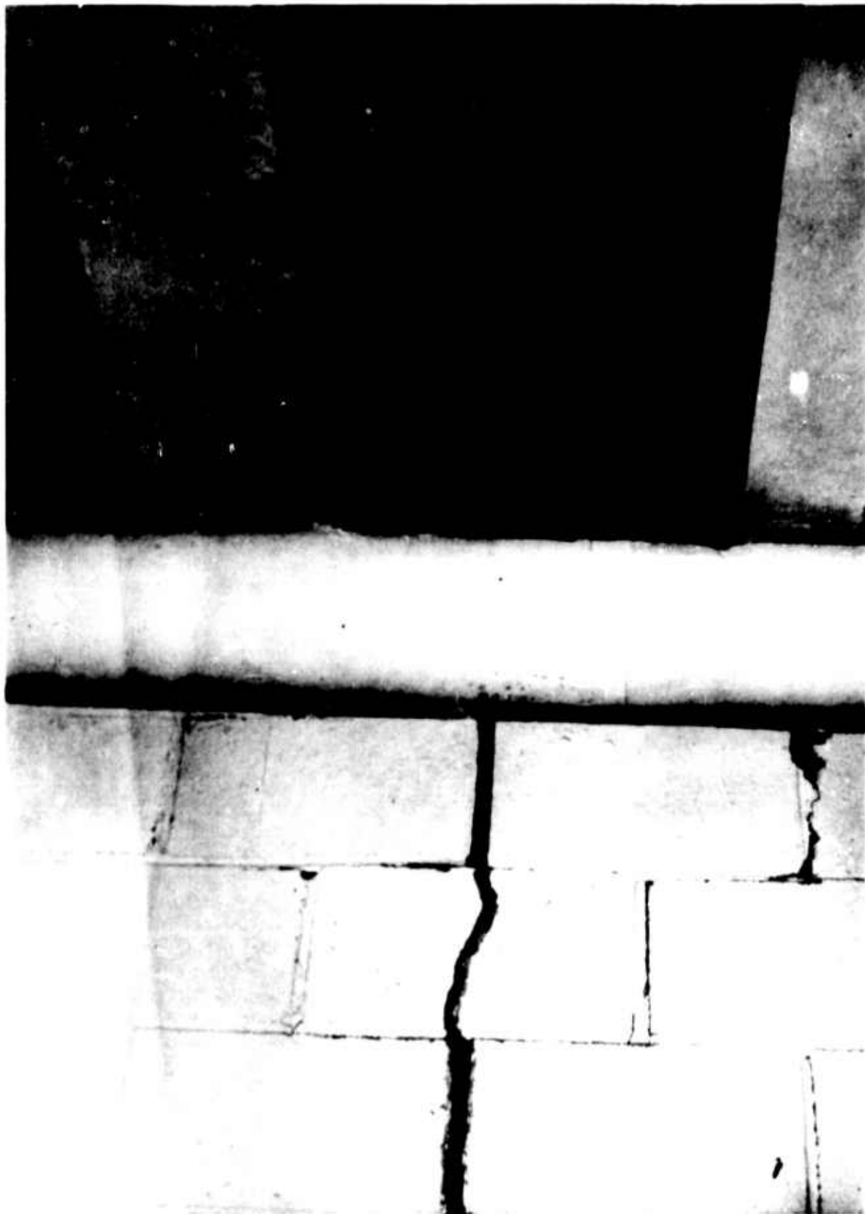
Figure 268. Elmendorf AFB Building 6-900 (Cracked masonry-block wall inside building)
