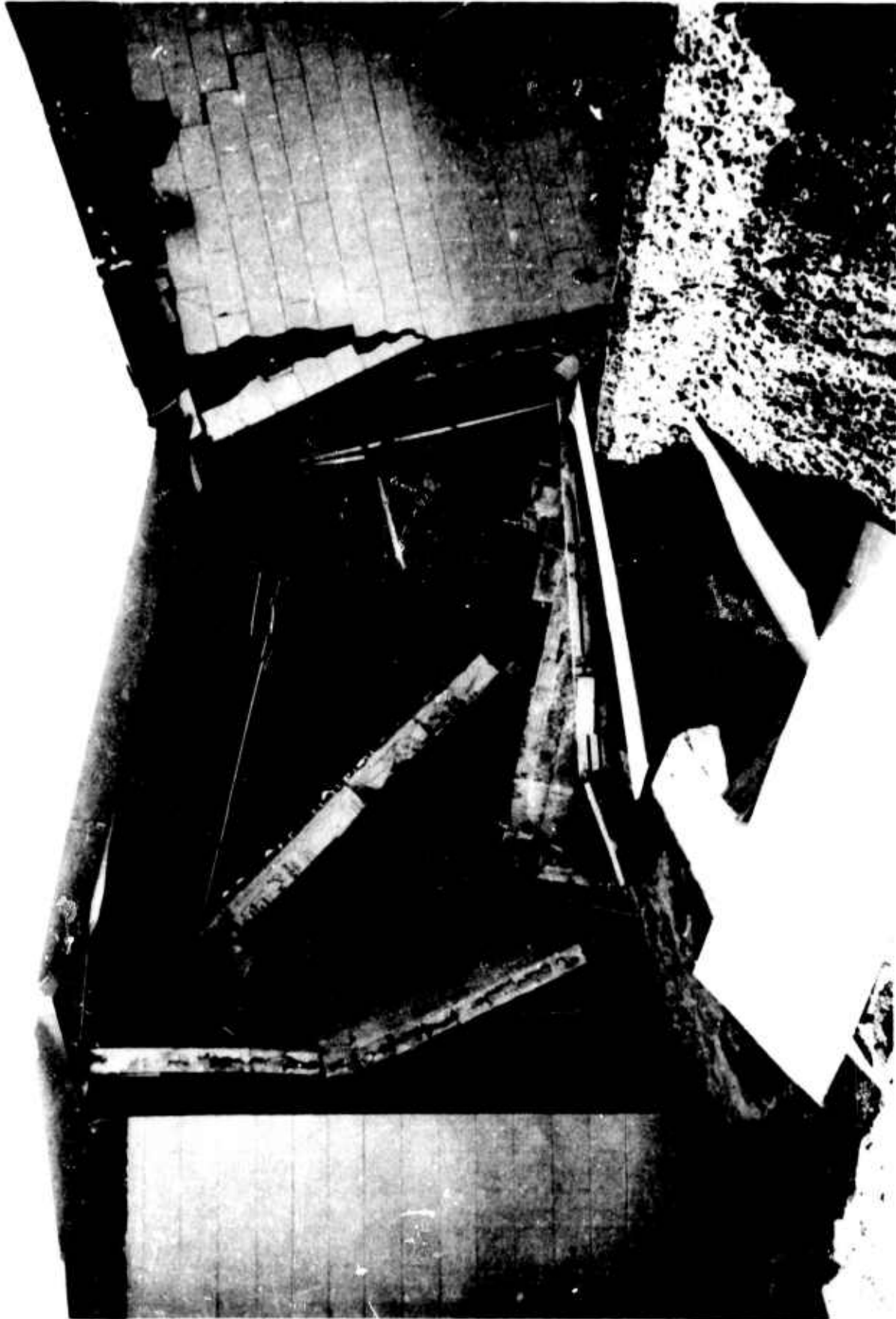
Figure 101. Government Hill Slide (Looking into the east-west corridor of the Government Hill school)
