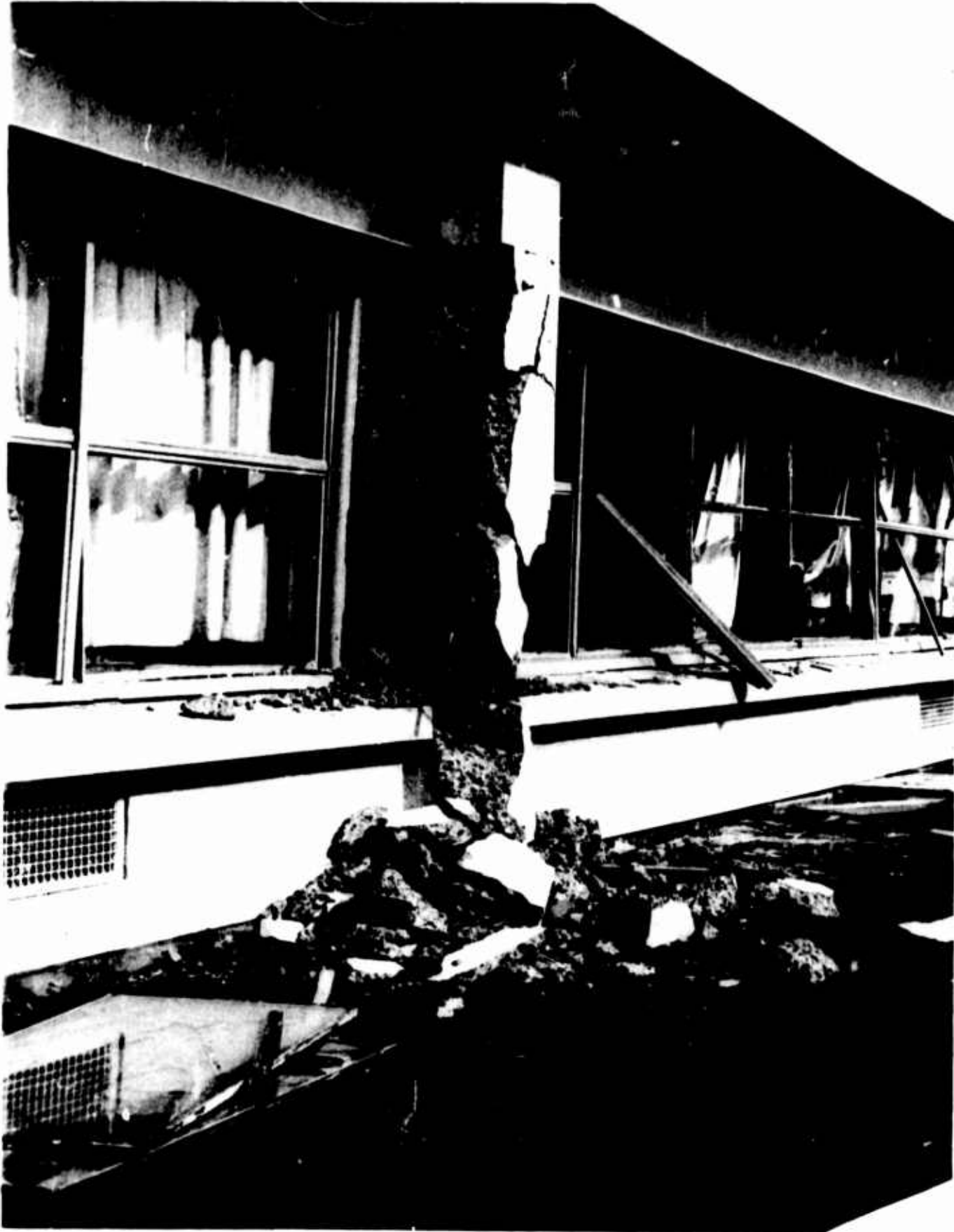
Figure 182. West Anchorage High School (Damage to short second-story column in south wall of wing B above the cafeteria was not prevented by light horizontal ties)
