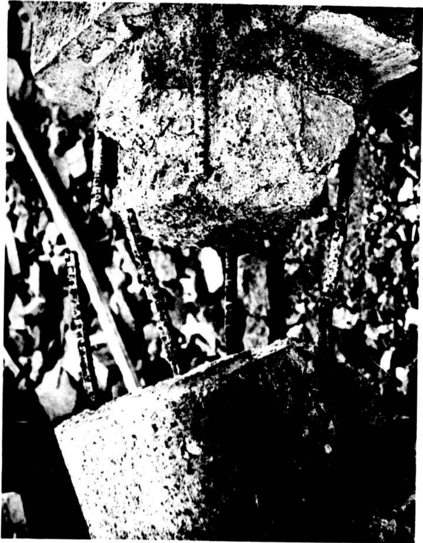
Figure 206. Gay Airways Hangar (Closeup of fractured pilaster rebar overlap)
