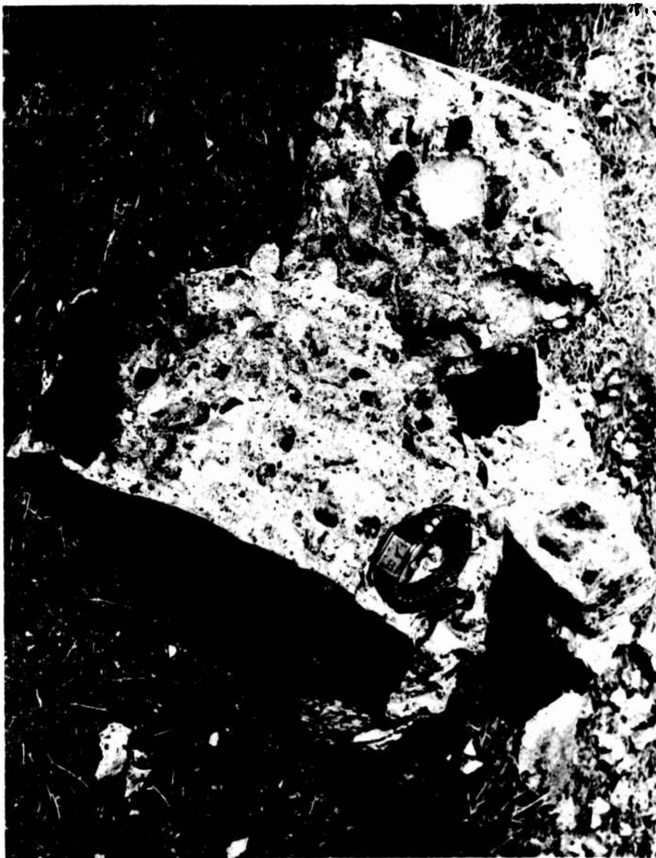
Figure 265. Elmendorf AFB Field House (A fallen piece of concrete from southwest corner of gymnasium showed few aggregate fractures)
