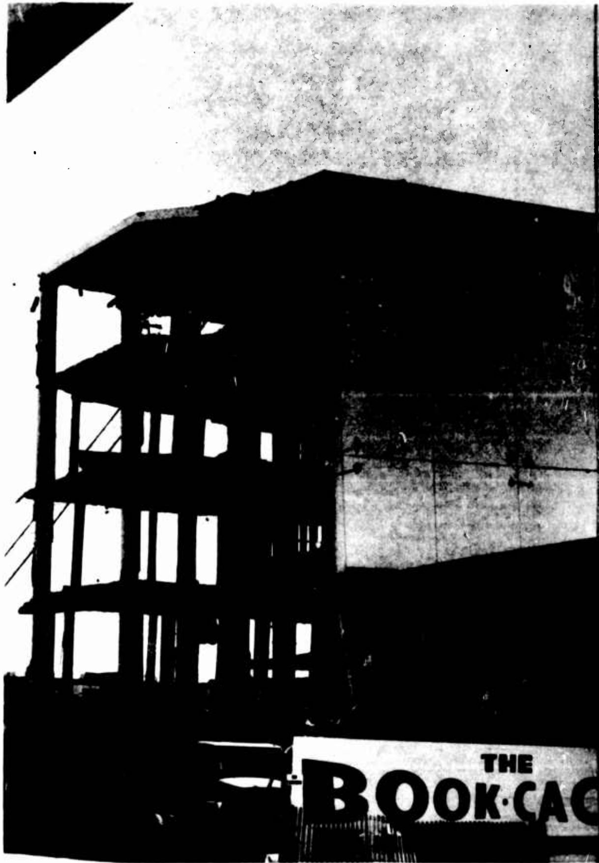
Figure 143. J. C. Penney Building (Floor slab failures along the north side of the structure)
