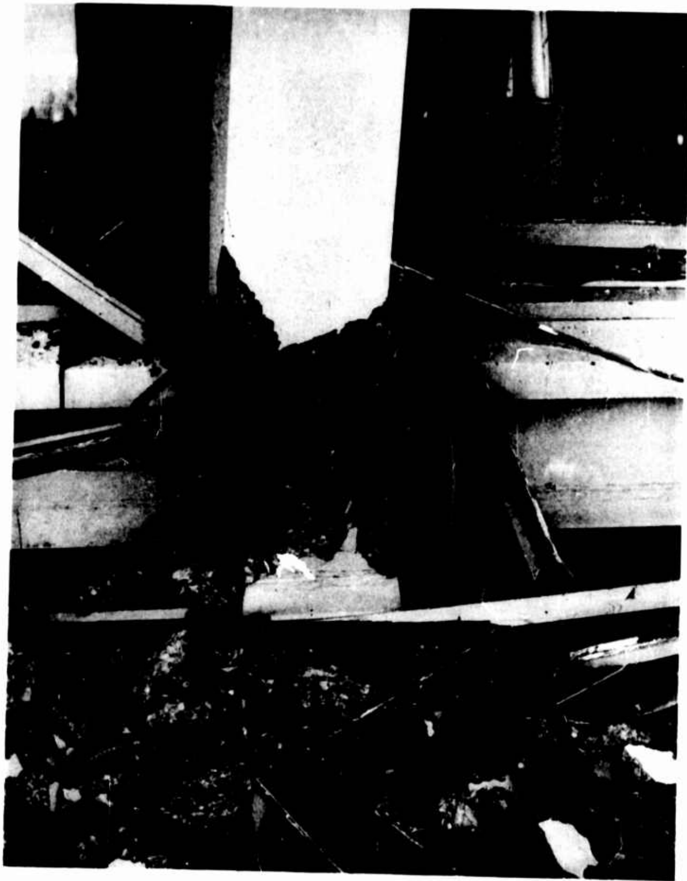
Figure 178. West Anchorage High School (Closeup of the base of the column shown in figure 177)
