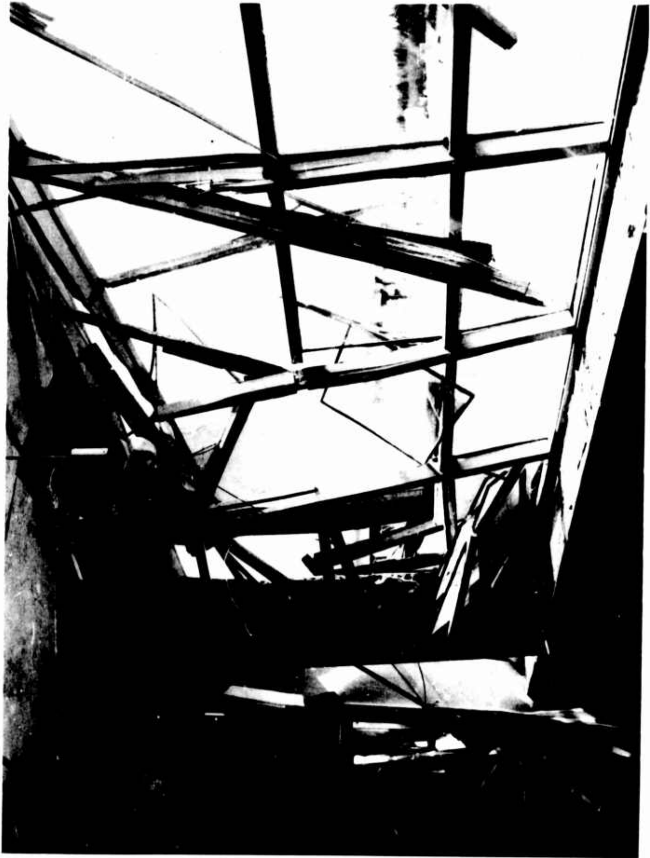
Figure 184. West Anchorage High School (Interior damage to second-floor classroom on south side of wing B)
