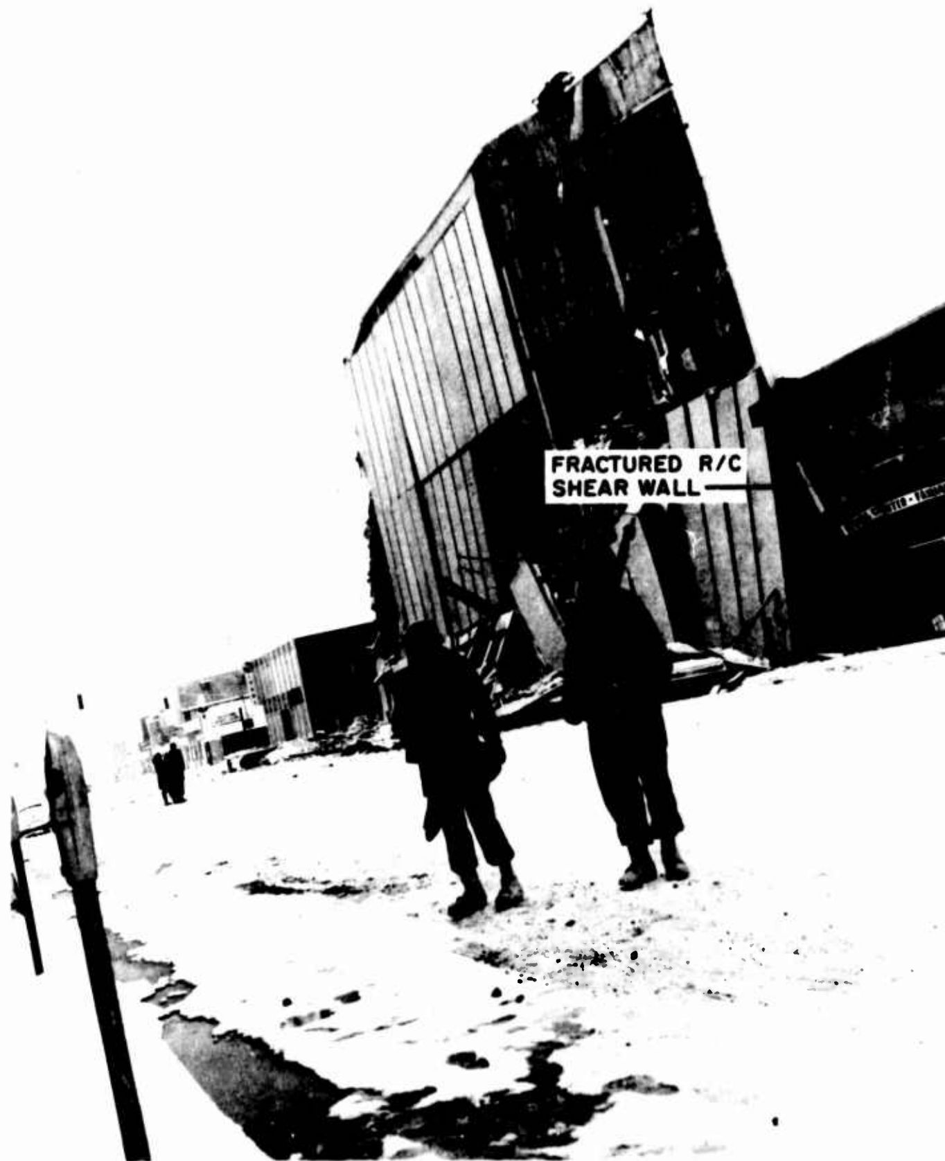
Figure 137. J. C. Penney Building (Fallen precast reinforced-concrete curtain wall panels along the north side of the structure)
