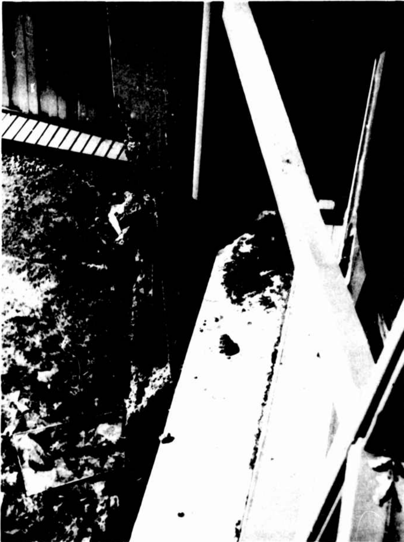
Figure 181. West Anchorage High School (No horizontal ties are visible at the base of the column shown in figure 180)
