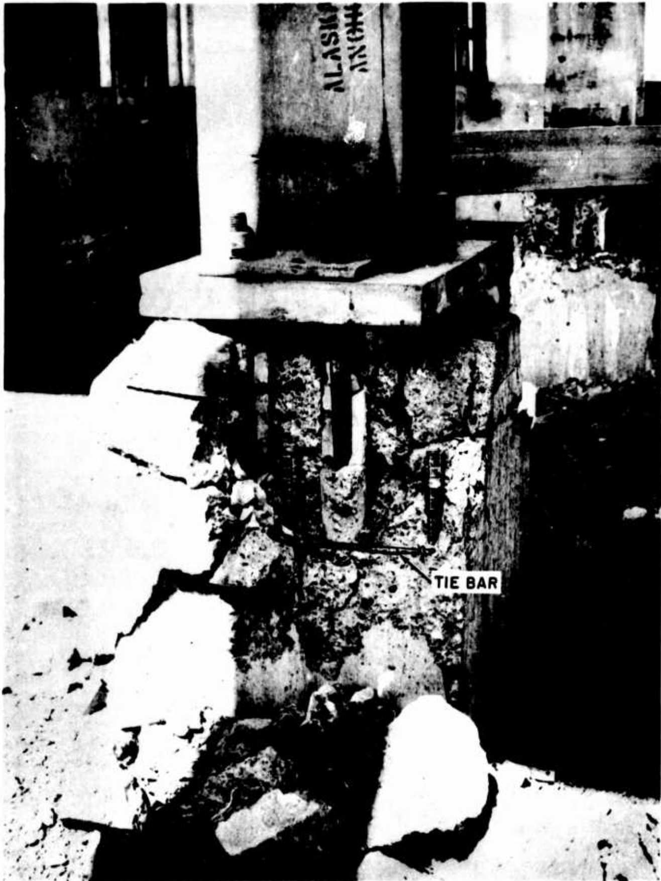
Figure 224. Alaska Brewery Company Structure (Damage to an interior footing, mainly above first horizontal tie)
