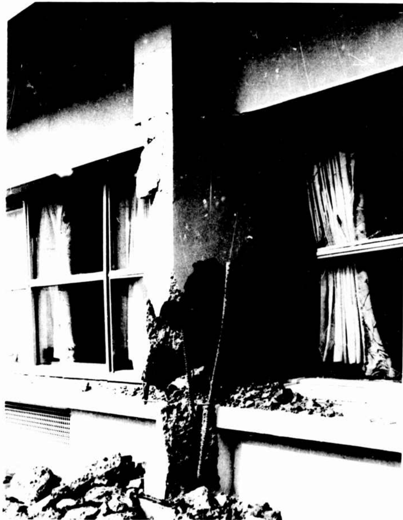
Figure 183. West Anchorage High School (The other side of the column shown in figure 182)
