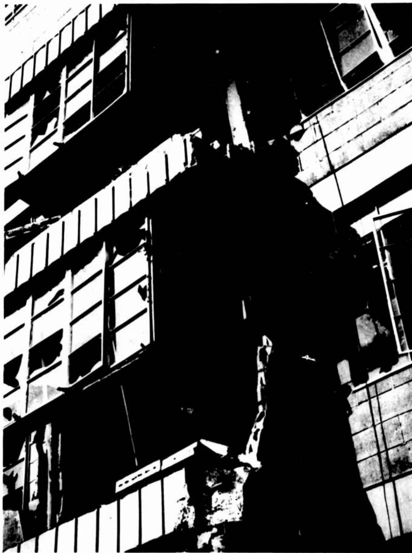
Figure 277. Hillside Apartments (Window frames in rear of building remain suspended from steel beams after masonry-block walls around them fell)
