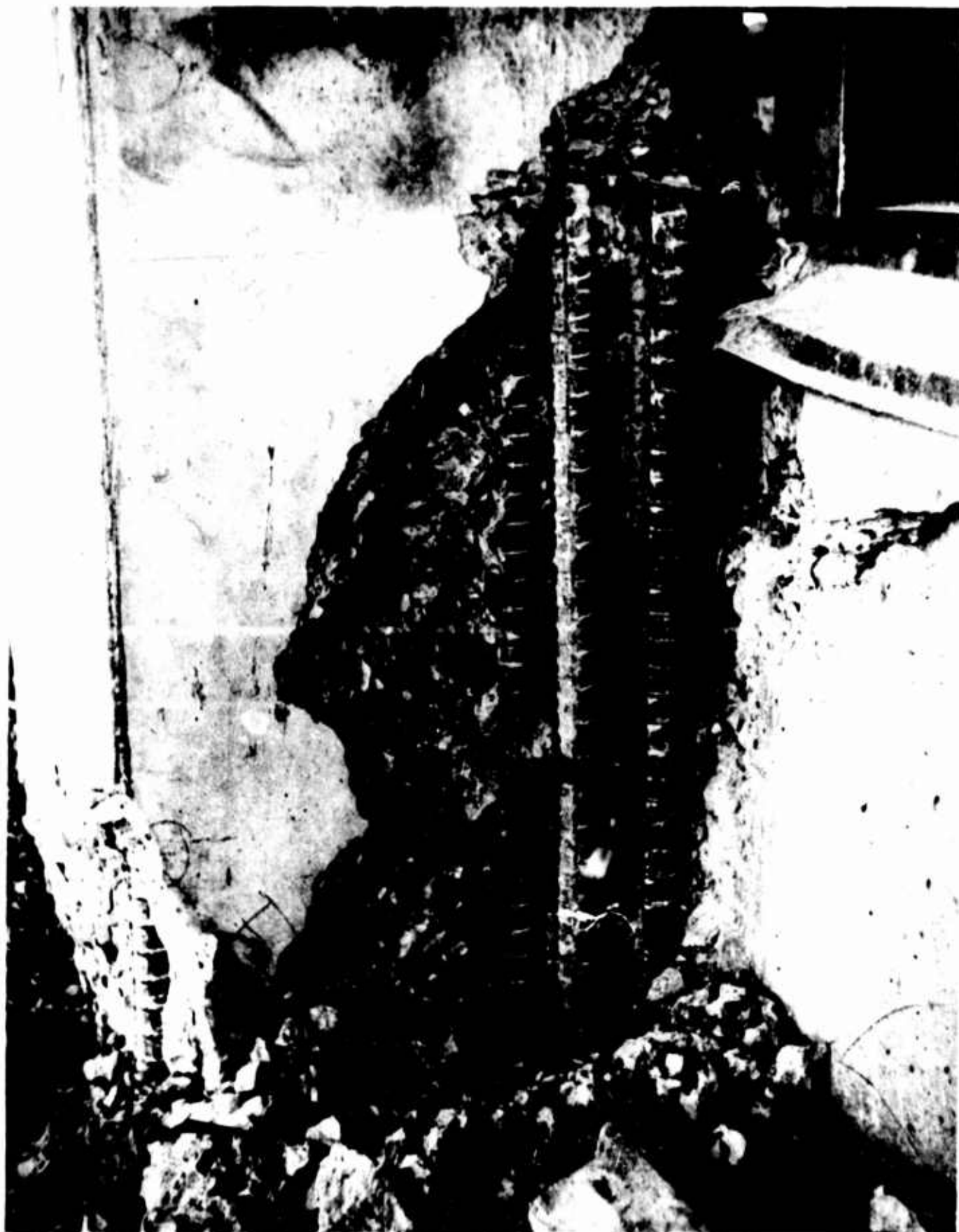
Figure 210. Alaska Sales and Service Building (Spalling at the base of a heavy T-column along the north side of the structure)
