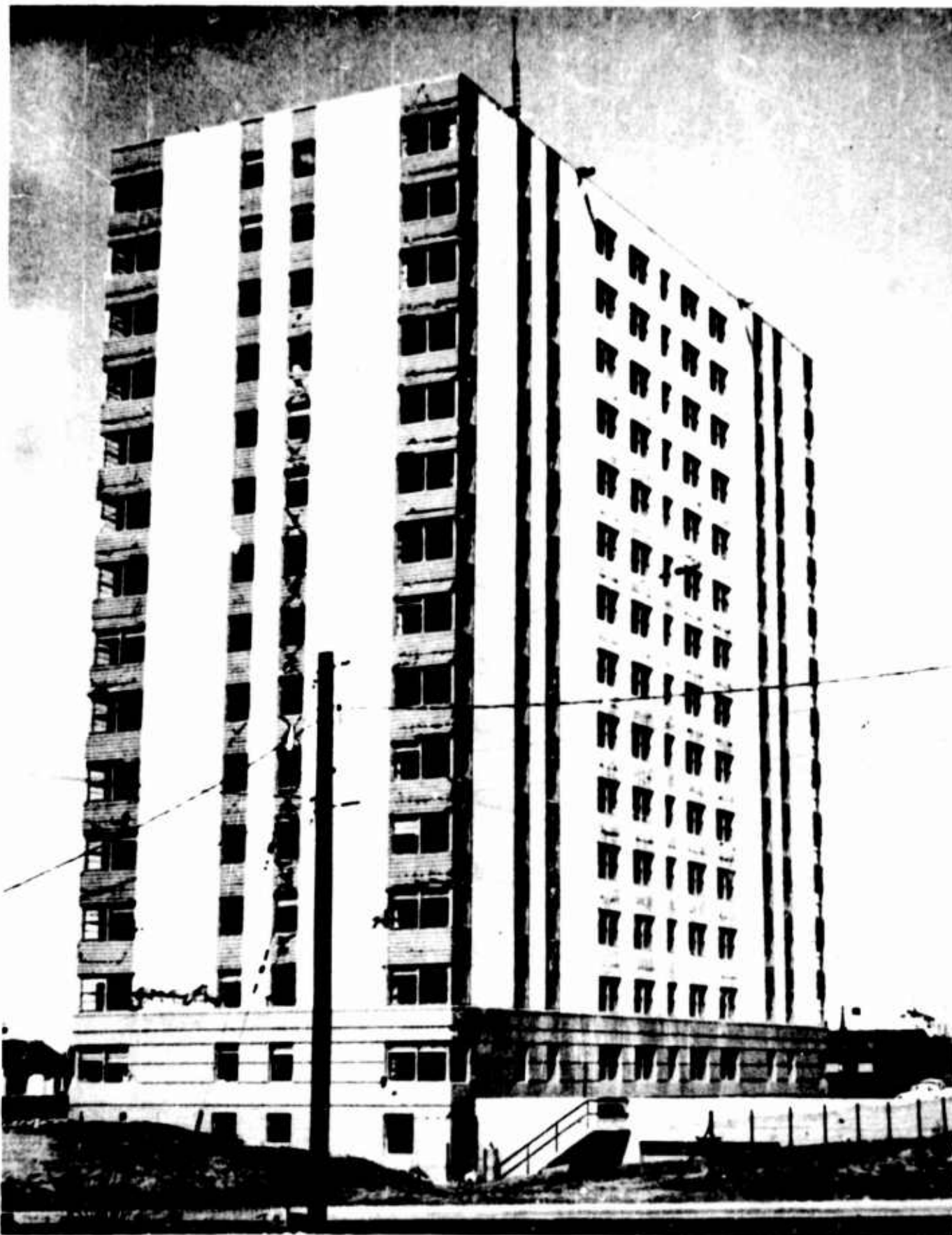
Figure 147. Twelve-Hundred L Street Apartments (South side of the structure showing column wall fracture midway between the second- and third-floor levels)
