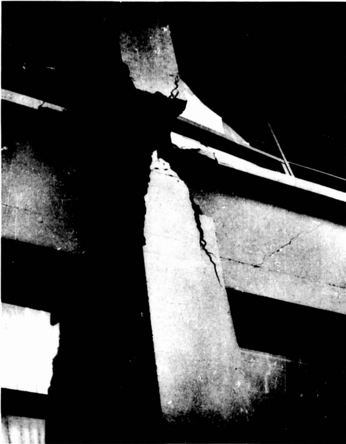
Figure 175. West Anchorage High School (Closeup of damaged column shown in figure 174)
