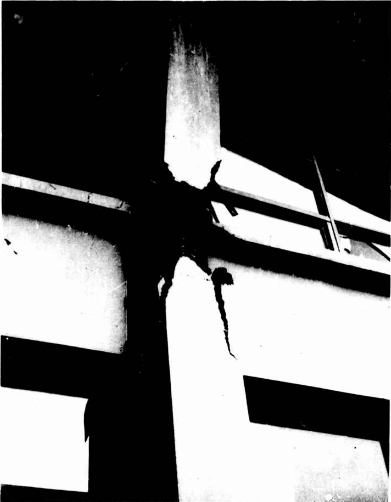
Figure 176. West Anchorage High School (Closeup of damaged column shown in figure 174)
