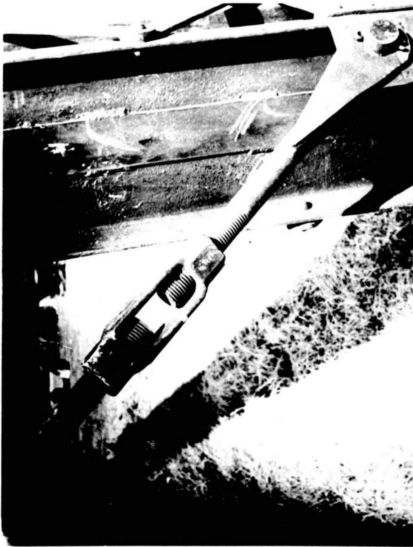
Figure 251. Alaska Native Hospital Water Tower (Tie-rod turnbuckle at base of tower shows no sign of yielding)
