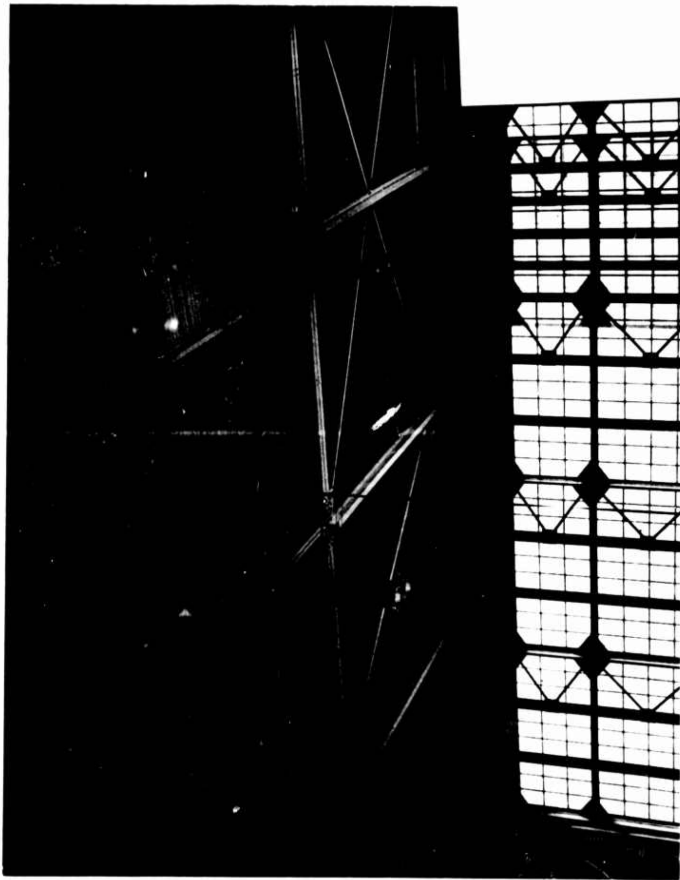
Figure 211. Elmendorf AFB Aircraft Maintenance Hangar (Roof framing in the hangar)
