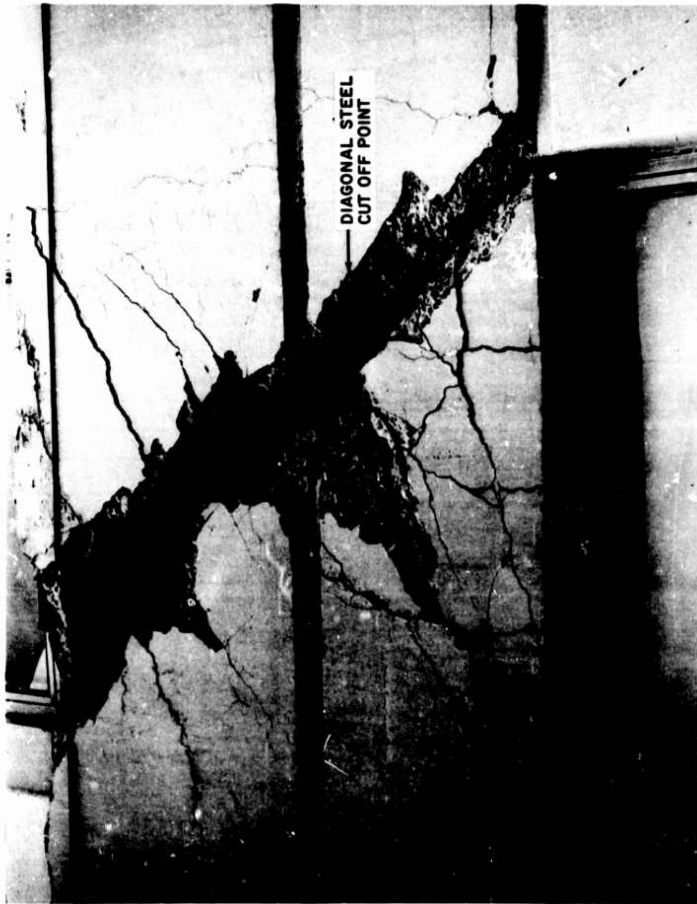
Figure 153. Mount McKinley Building (Diagonal tension failure in east wall at second-floor level)
