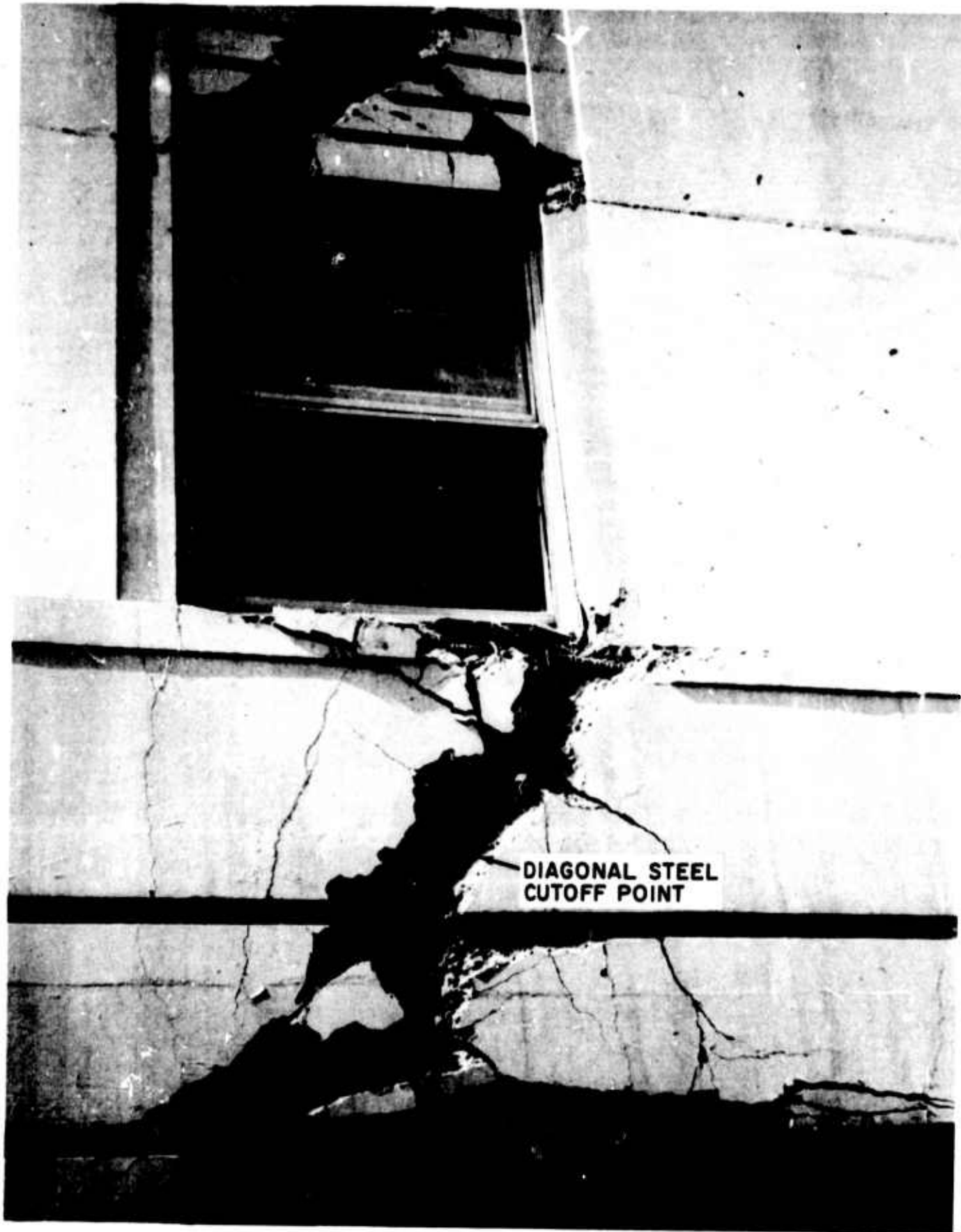
Figure 152. Mount McKinley Building (Diagonal tension failure in east wall at second-floor level)
