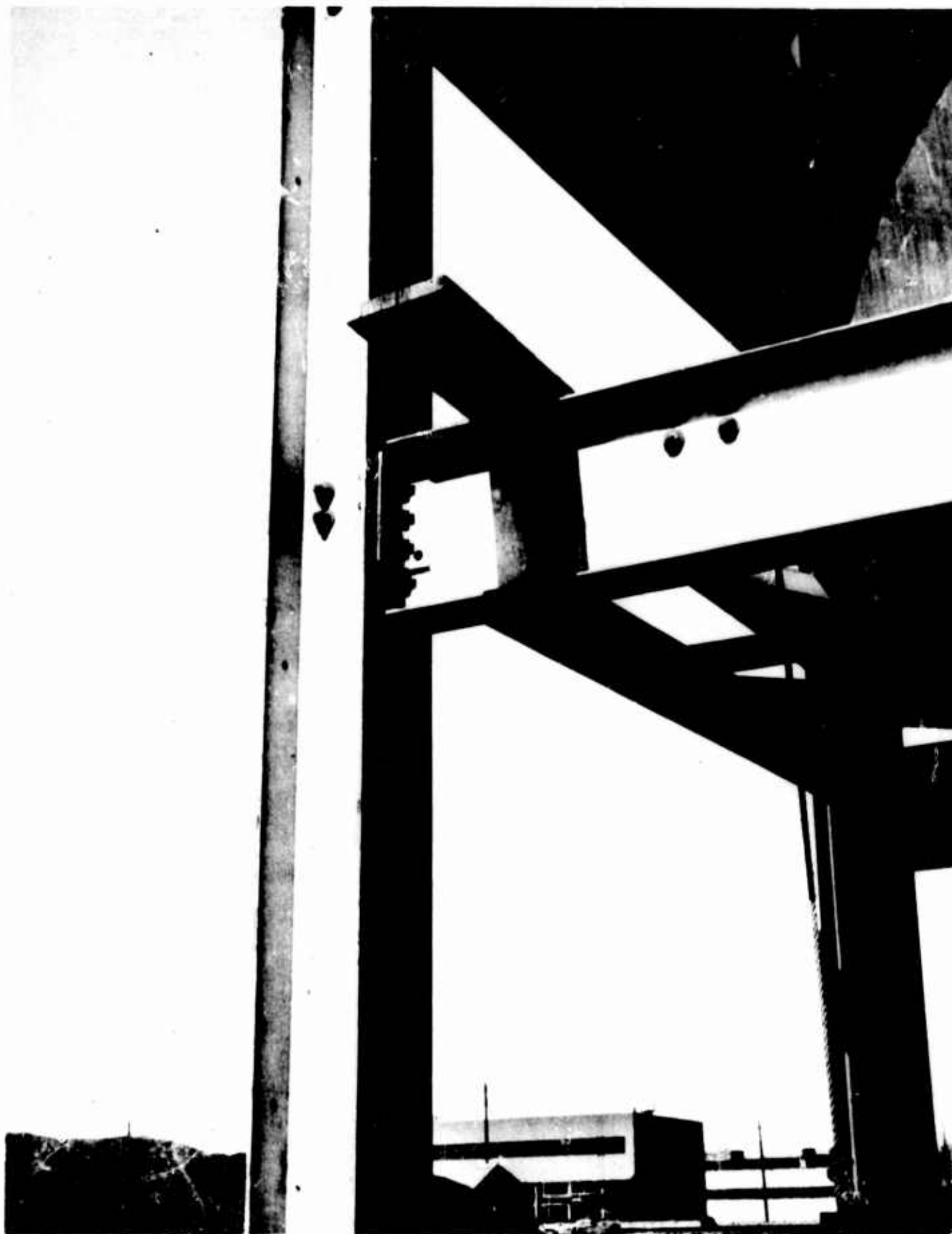
Figure 222. Alaska Brewery Company Structure (Typical undamaged bolted connection)
