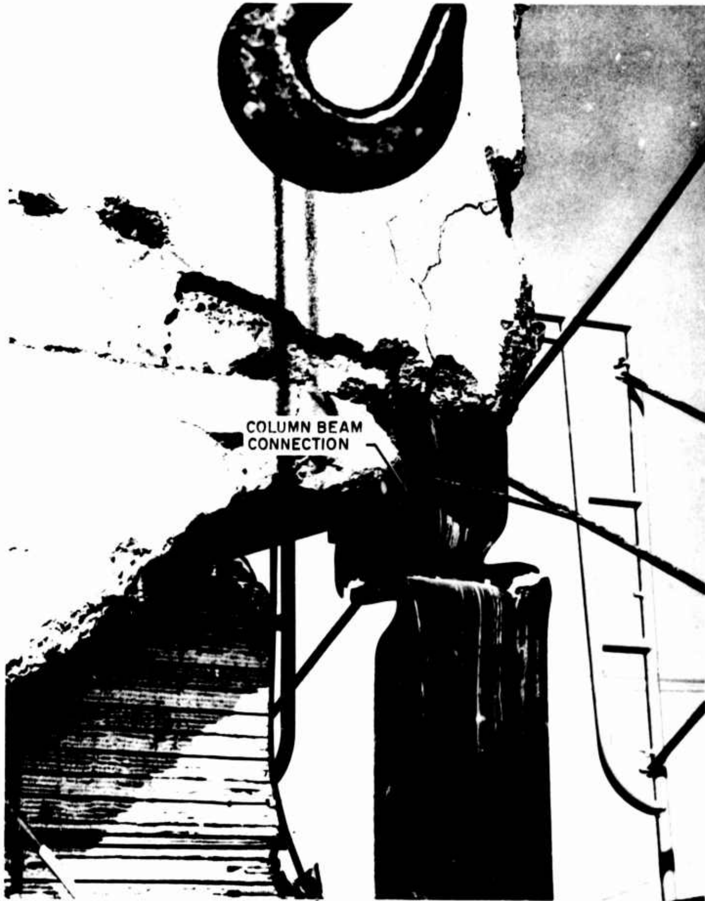
Figure 219. Cordova Building (Shear buckle in southeast corner column of building)
