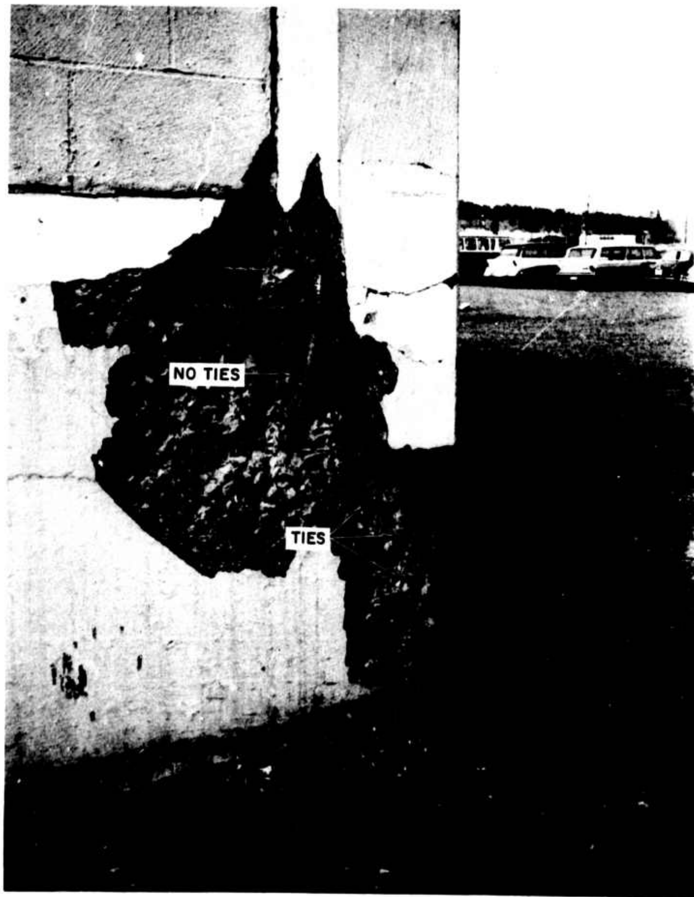
Figure 126. Elmendorf AFB 750-Man Barracks (Column shear failure at first-floor level in northeast corner of Building 31-250. Notice absence of ties in failure zone.)
