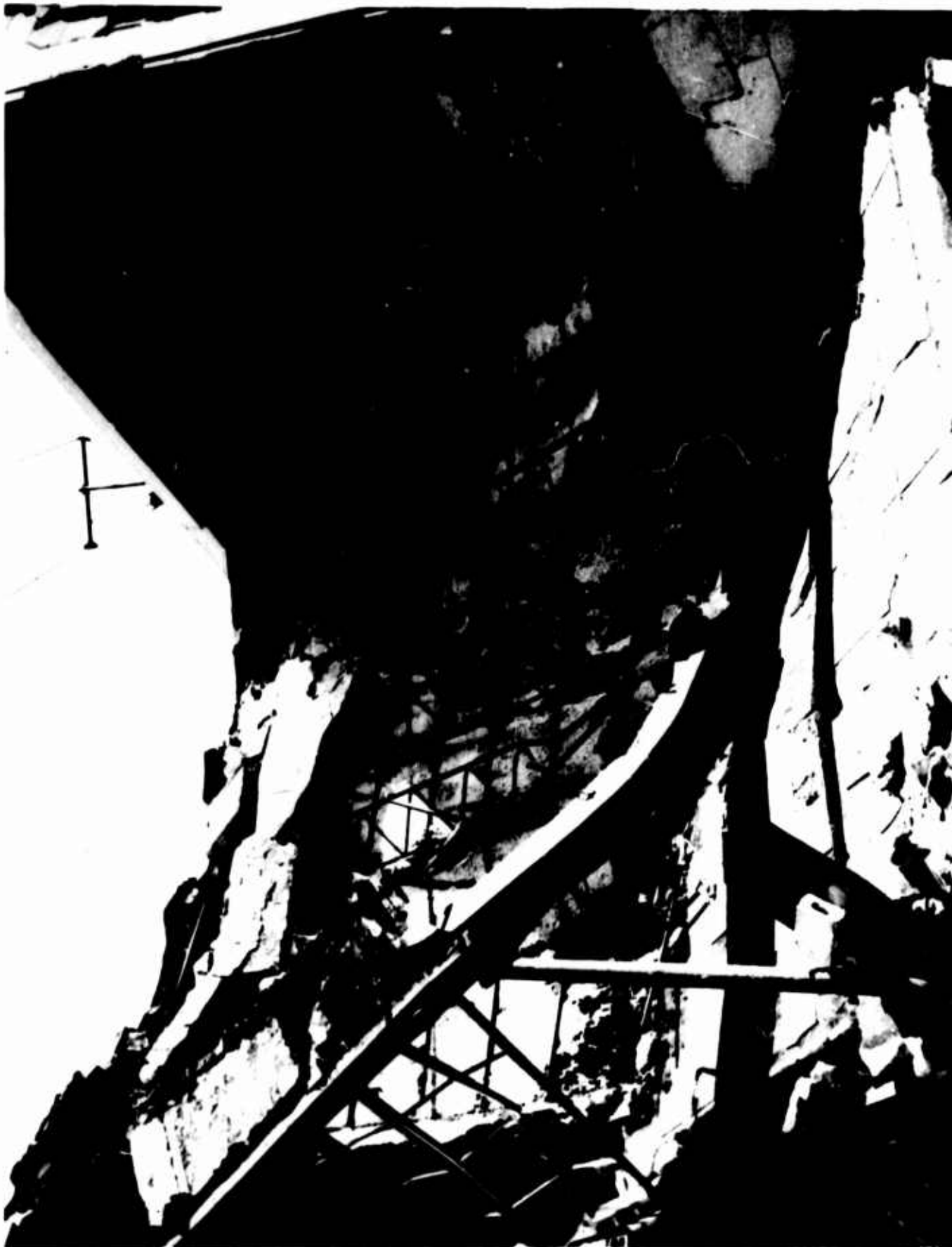
Figure 276. Hillside Apartments (A masonry-block partition near northwest corner of building fell without cracking more than a few blocks)
