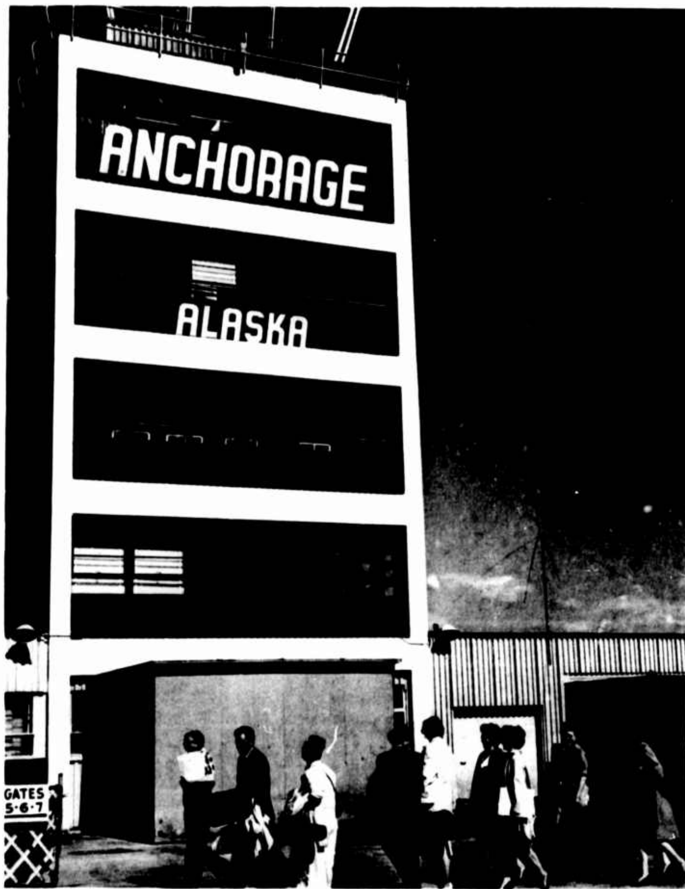
Figure 134. Anchorage international Airport Control Tower (Before the earthquake)
