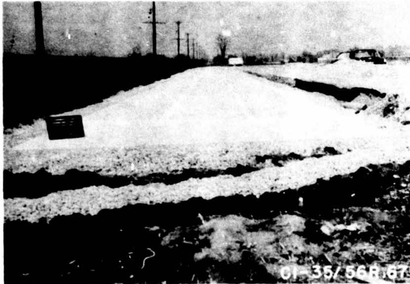
Part 1 - Ready for Traffic Looking North
