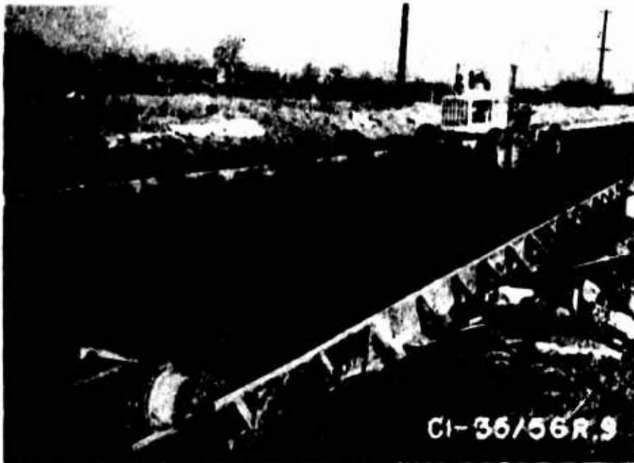
Grading Operations - Part 1
