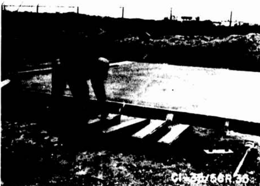
Field Beams for Laboratory Testing Part 1
