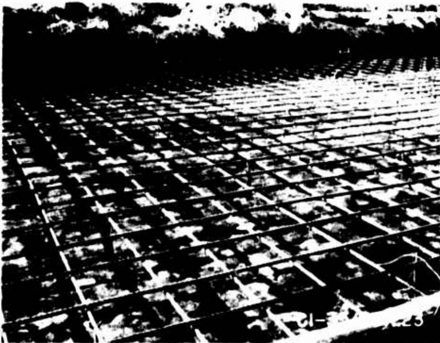
Reinforcing Steel in Place, Item 55 Part 1, #5 on 12-Inch Centers
