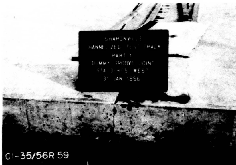
Controlled Cracking at Dummy Groove Contraction Joint - Part 1
