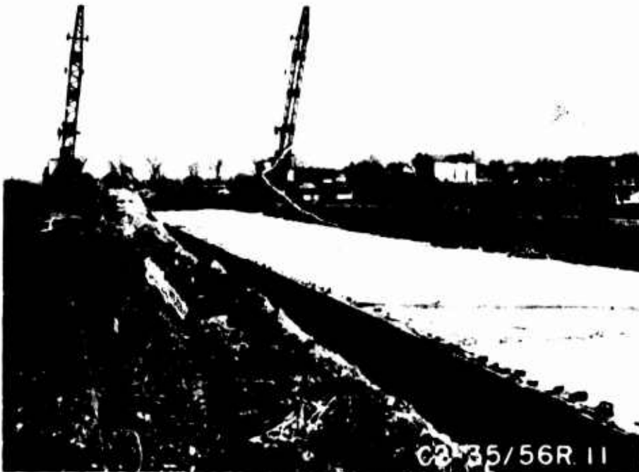
Part 2 - Ready for Concreting at North End
