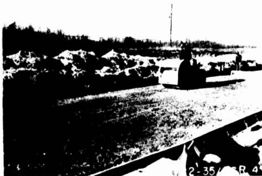
Grading Operations - Part 2
