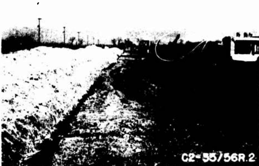
Part 2 - Subgrade, Looking North
