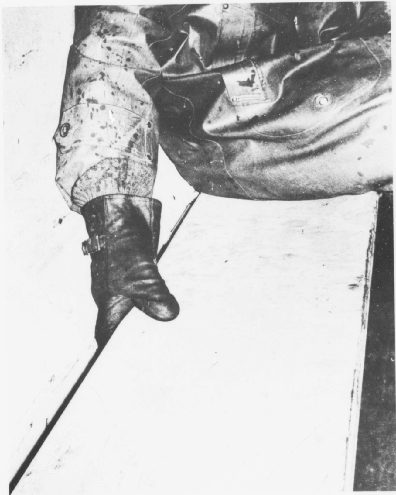
FIG 8. The space between the bench and the wall in the personnel compartment is apt to catch items such as the shovel.
