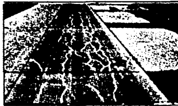
6" CONCRETE ON 6" COMPACTED SAND AND GRAVEL ON 66" SOIL STABILIZED SAND AND GRAVEL SLAB S2.66
