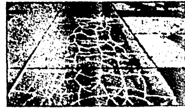
6" CONCRETE ON 12" COMPACTED SAND AND GRAVEL ON 60" SOIL STABILIZED SAND AND GRAVEL SLAB R2.612
