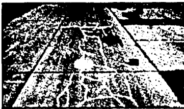
6" CONCRETE ON 12" COMPACTED SAND AND GRAVEL ON 60" SOIL STABILIZED SAND AND GRAVEL SLAB R2.612
