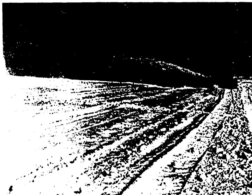
Figure 9. Aerial delivery of fill snow with a tractor-mounted snowplow.
