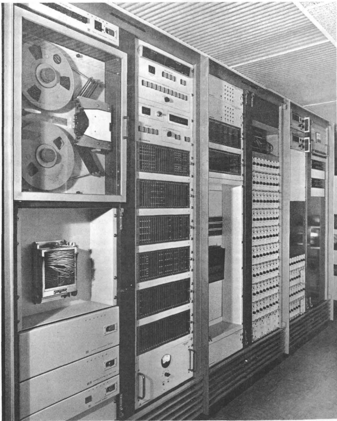
FIG. 5 - DIGITAL DATA ACQUISITION SYSTEM IN VAN
