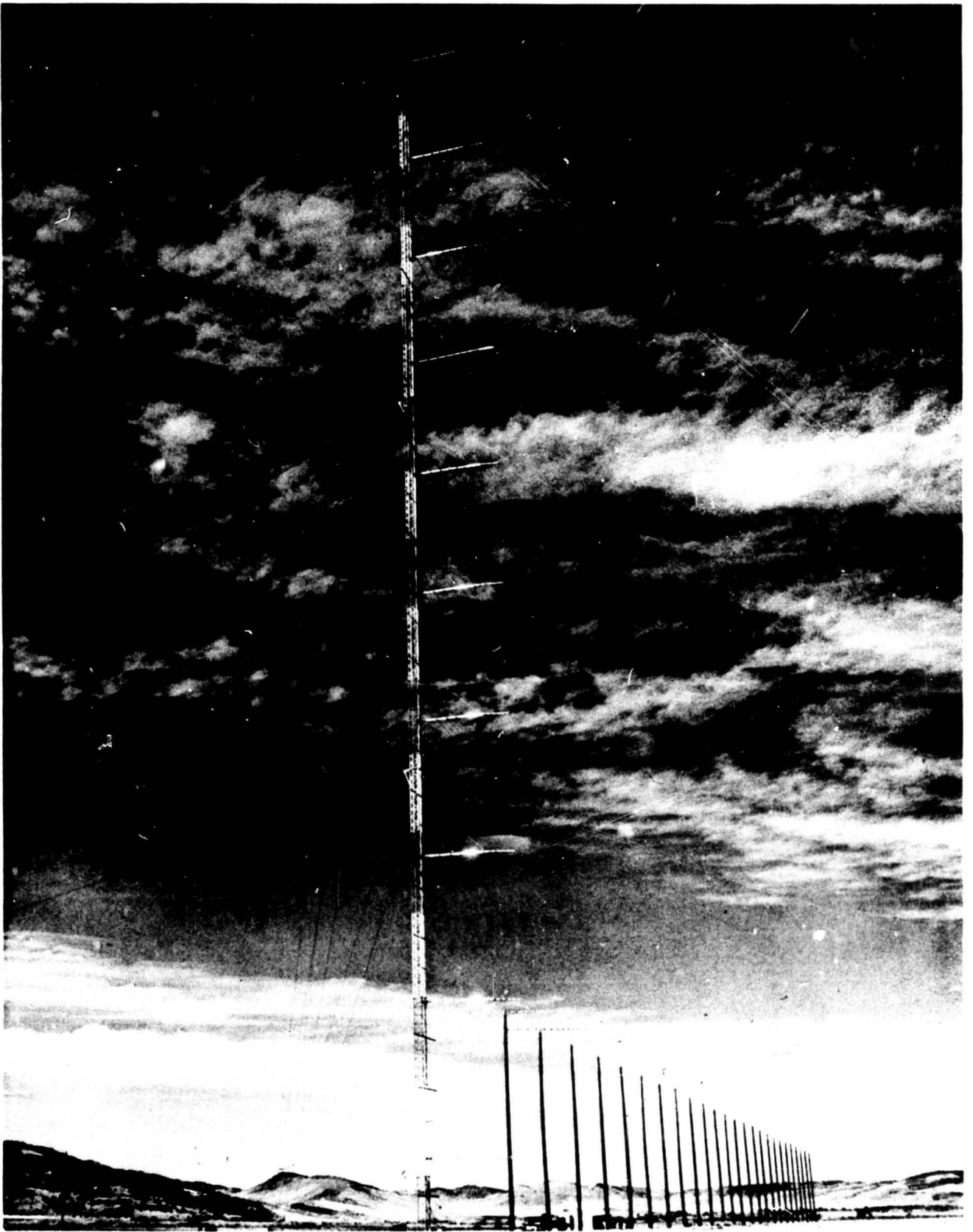
Figure 1 The elevation-scan array and the adjacent azimuth-scan array.
