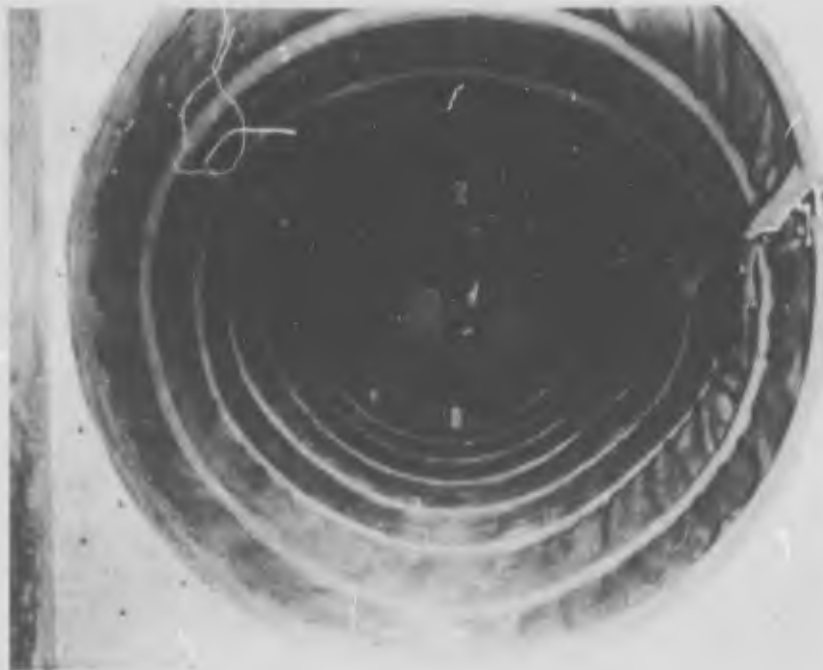
Fig. 20. Ring deflections at 6-ton level (note testman in background taking vertical deflection measurement of Ring No. 6)
