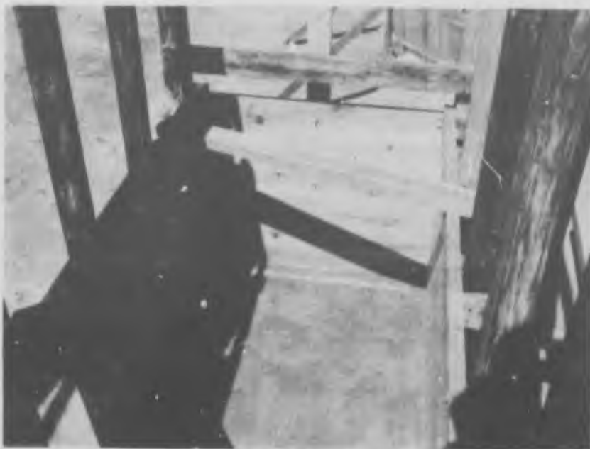
F8077 Fig. 11. Sand in top bearing struck off level at an elevation 6 inches above liner crown.
