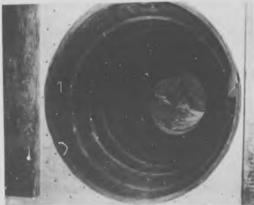
Fig. 10. Ring joints oriented on horizontal diameter to right side of vertical axis; excess webbing covering joints.
