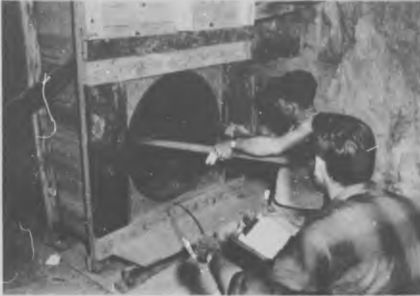
Fig. 14. Five-foot-length, field-constructed calipers inserted into liner to determine deflections.
