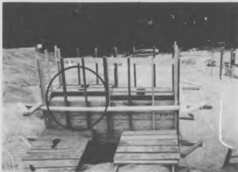
Fig. 18. First 2-ton surcharge (note left corner of timber top bearing plate).
