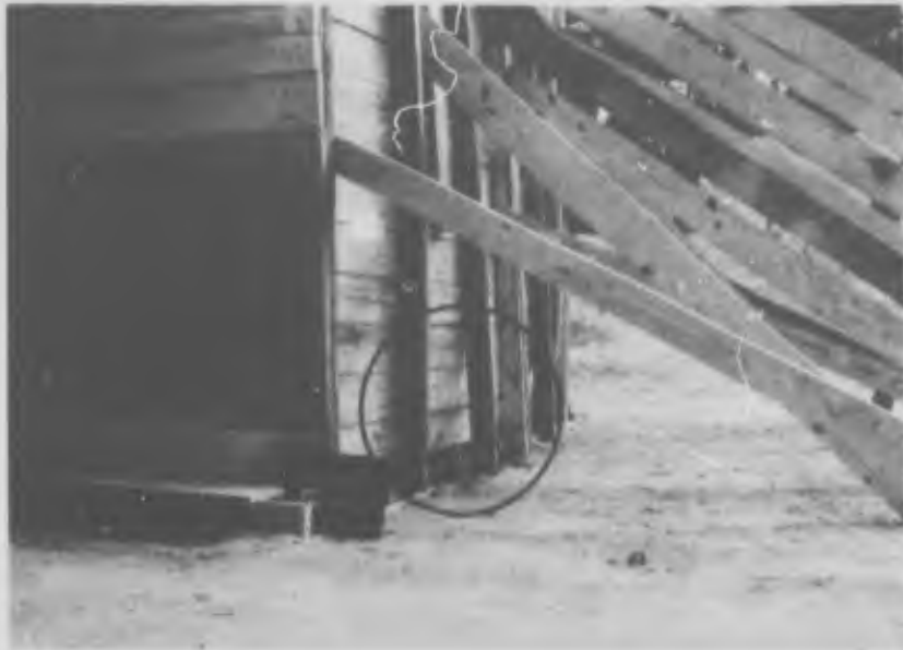
Fig. 27. North end of sandbox (note condition of wall panel studs).
