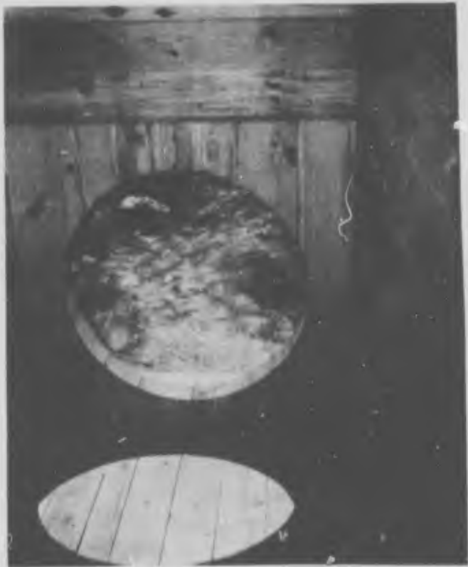
Fig. 5. Anchorage bulkhead was fabri- cated of 6 three-by- eights 42 inches long.
