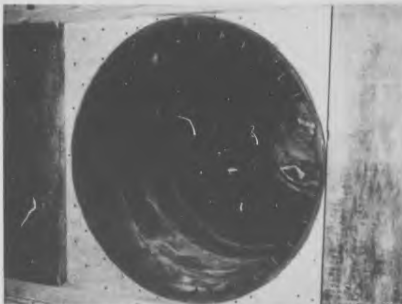
Fig. 8. Liner was secured to bulkhead by means of screws and washers through grommets affixed to liner.
