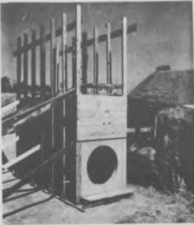
Fig. 4. Provisions for wall height extension.
