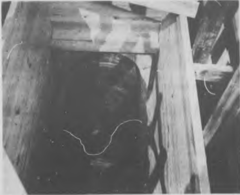
Fig. 9. Interior framing of bulkhead.
