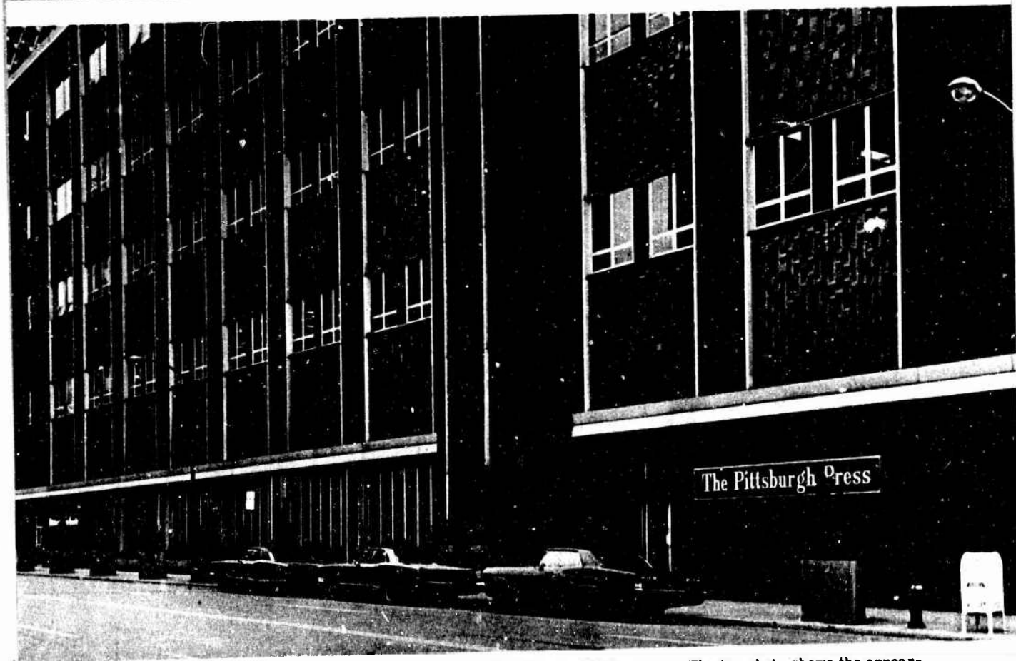
Figure 16.-Flood proofing at Pittsburgh Press Building. The top photo shows the appearance of initial flood proofing. The lower photo shows how the "face lifting" blended the flood proofed windows into the building design. (Photos by Pittsburgh Press.)
