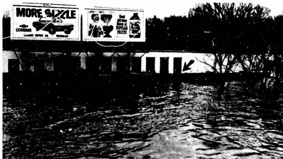
Figure 6.-Emergency Flood Proofing. Heavy planking covered over with polyethylene sheets (see arrow) was used to give emergency protection to this Waterloo, Iowa, plant during the April, 1965, flood on the Cedar River. (Photo by U. S. Army Corps of Engineers.)
