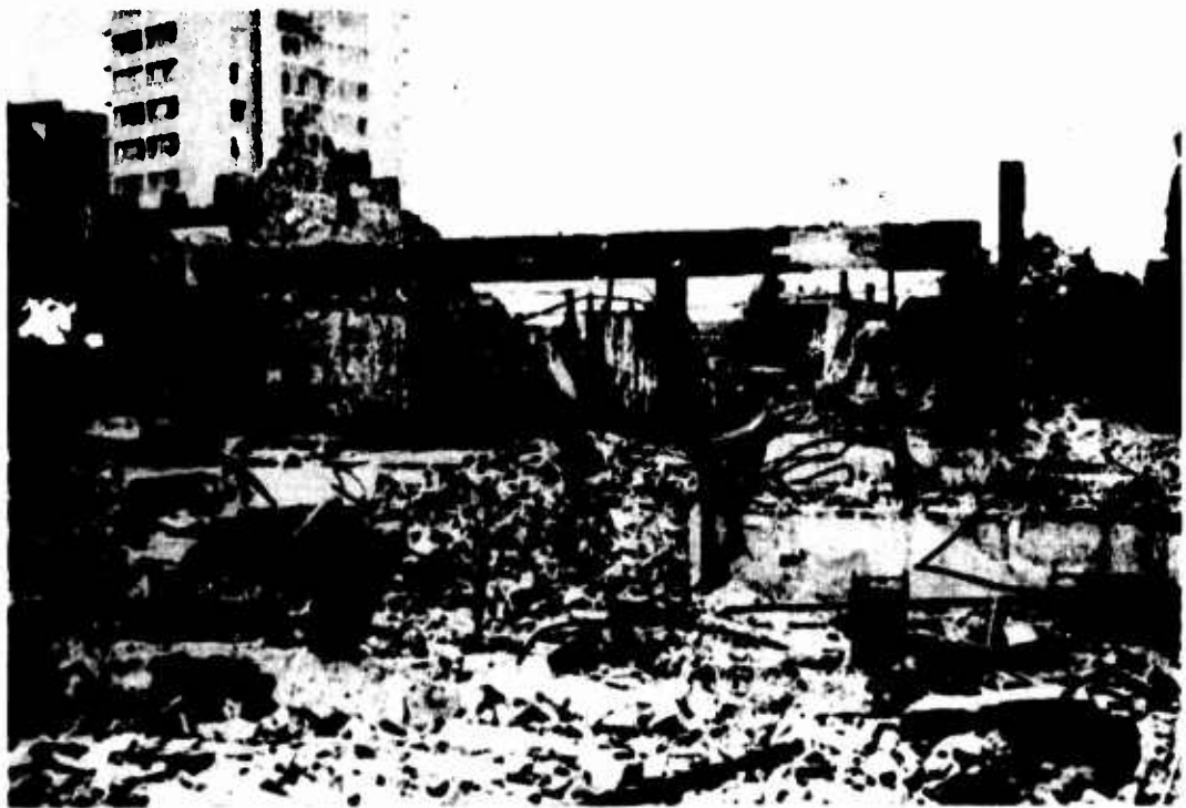
Picture 54 UNDAMAGED SKYSCRAPER SURROUNDED BY DEBRIS FROM FIRE-DAMAGED STRUCTURES
