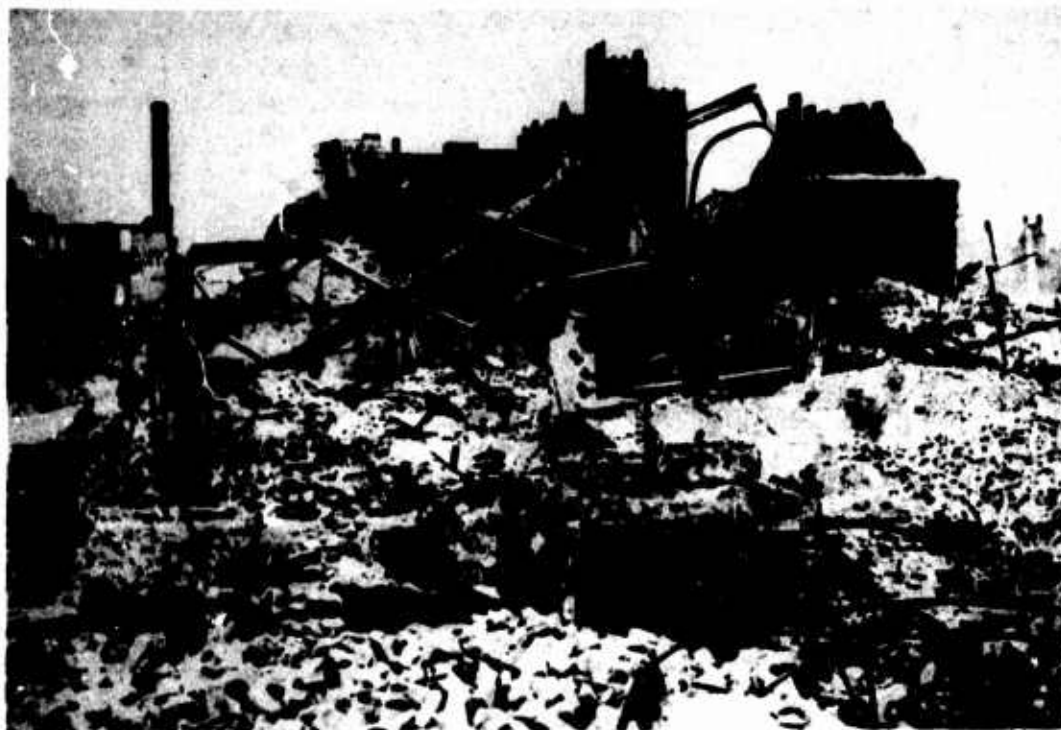
Pictures 37, 38 TWISTED STRUCTURAL STEEL, CHARACTERISTIC OF STRUCTURES DESTROYED BY FIRE
