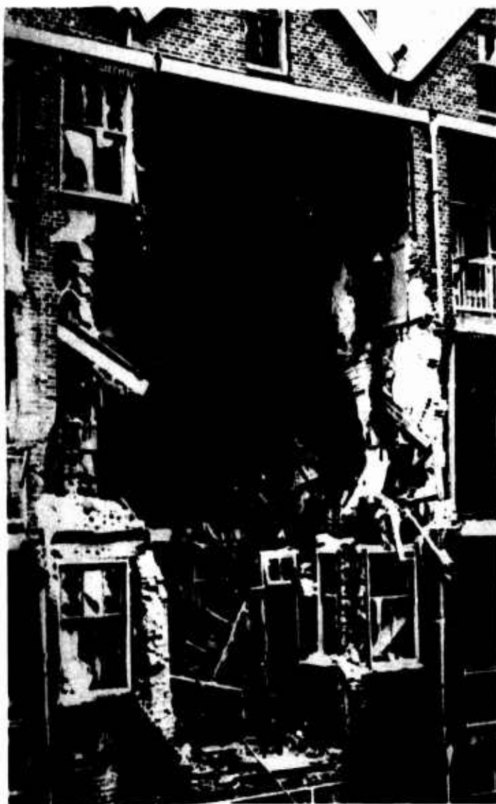
Picture 26 DIRECT HIT ON A RESIDENTIAL HOUSE. The bomb did not drop vertically through the roof but at an angle from above into the front wall of the house.
