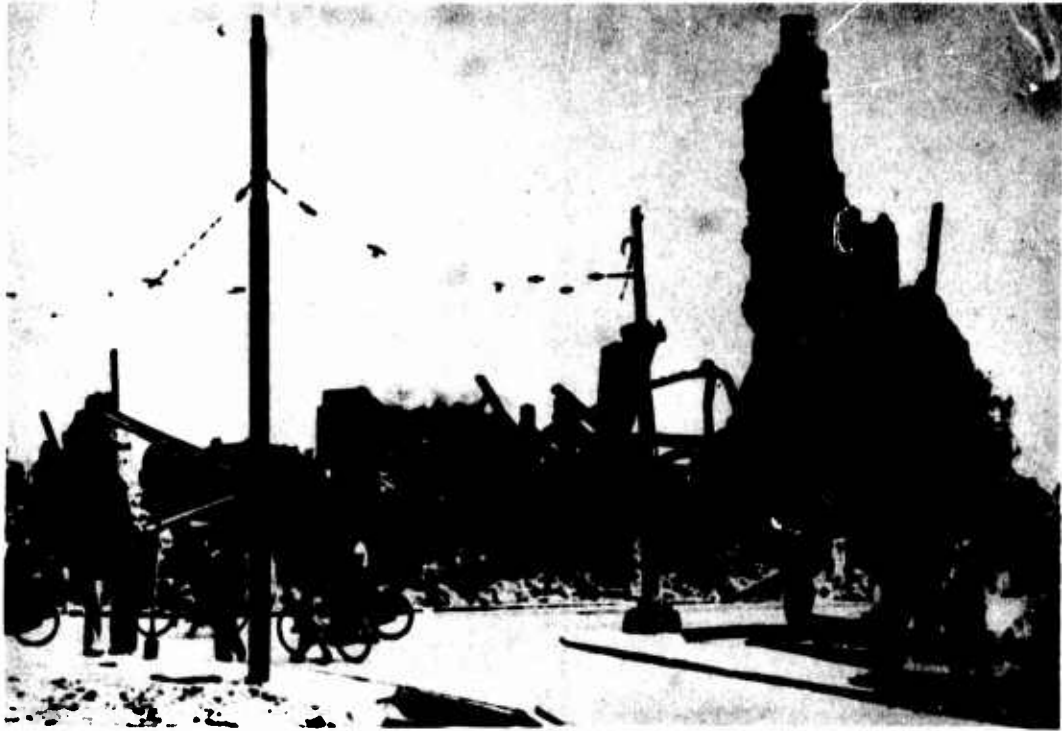
Figures 39, 40 TWISTED STRUCTURAL STEEL, CHARACTERISTIC OF STRUCTURES DESTROYED BY FIRE
