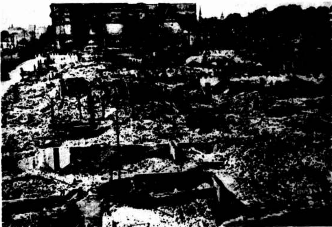
Pictures 31, 32 FIRE-DESTROYED STRUCTURES. All wooden parts, like beams, floors, doors, window frames, and shafts are completely burned. The fire sites are completely free of wood.
