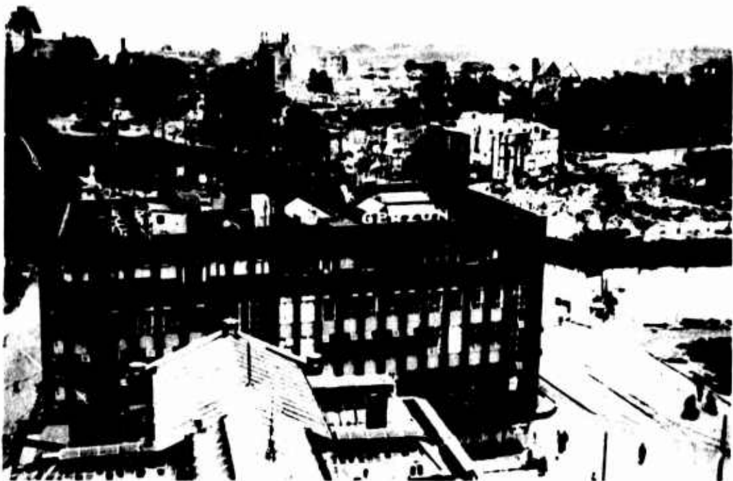
Picture 6 THE UNDAMAGED DEPARTMENT STORE GERZON AND THE GREAT MAAS BRIDGES IN THE BACKGROUND
