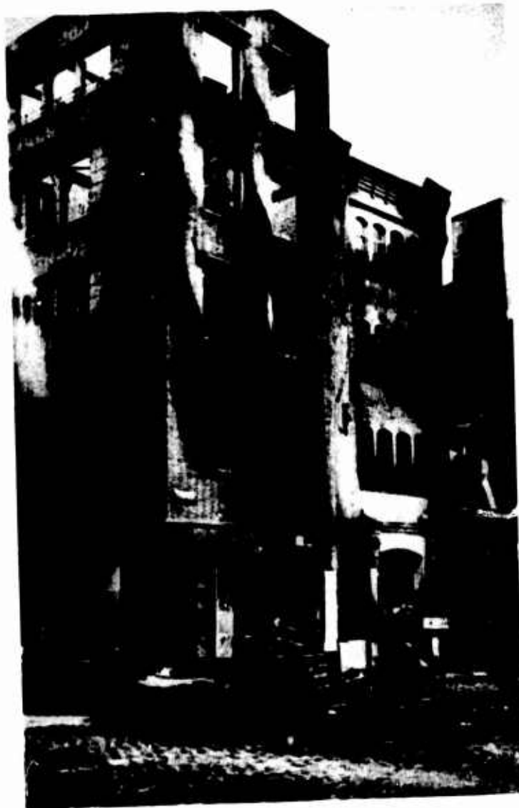
Picture 54 SOOT-BLACKENED STRUCTURE
