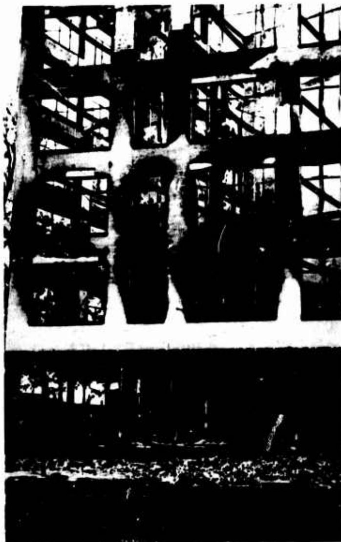
Picture 55 SOOT-BLACKENED STRUCTURE
