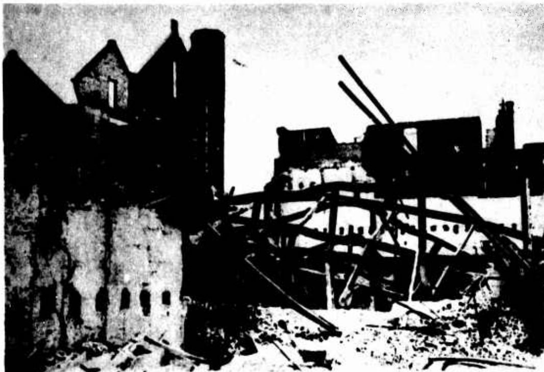
Pictures 37, 38 TWISTED STRUCTURAL STEEL, CHARACTERISTIC OF STRUCTURES DESTROYED BY FIRE
