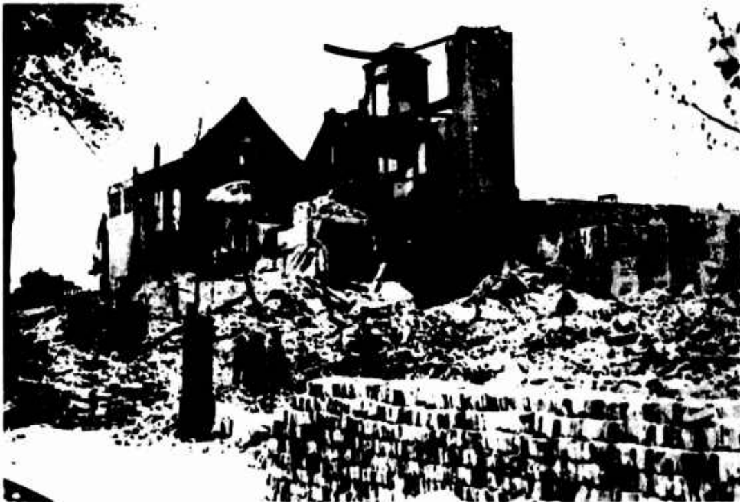
Picture 81 BRICK DEBRIS AFTER THE FIRE
