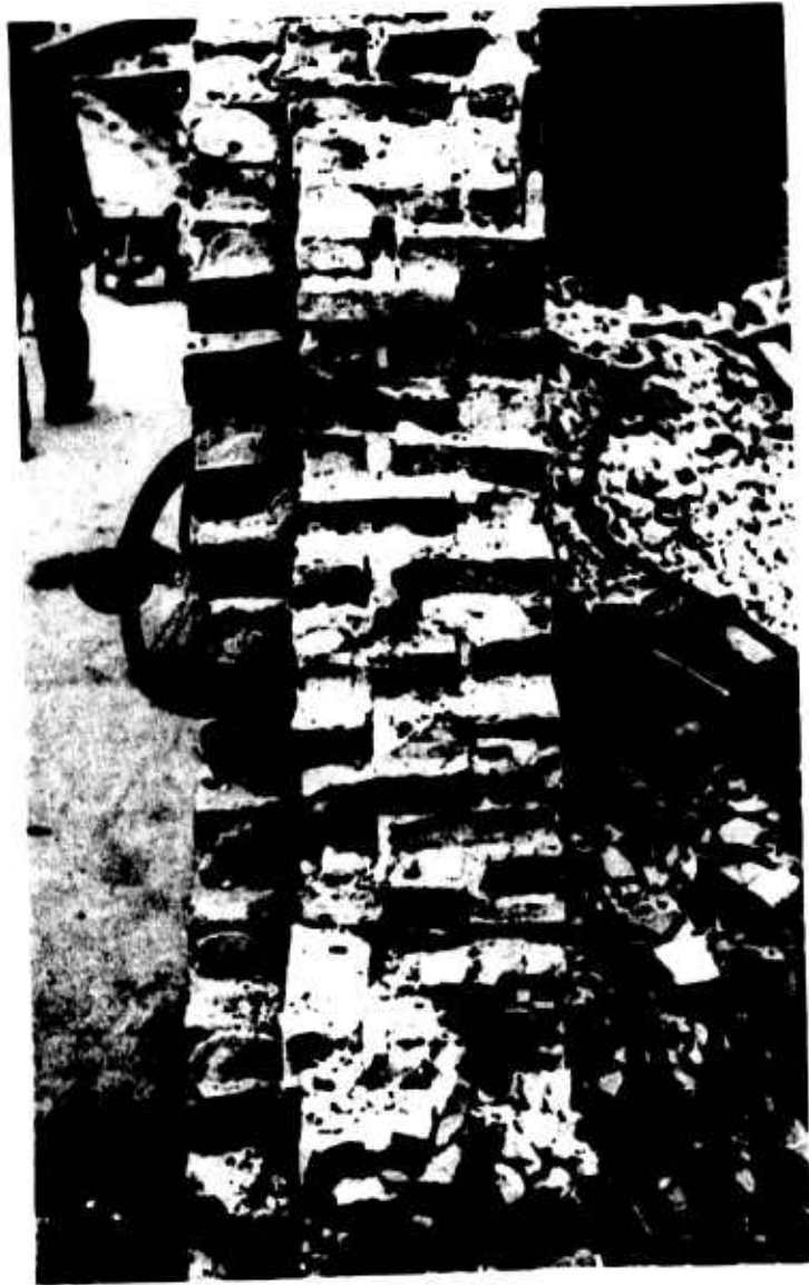
Picture 75 ILLUSTRATION OF DUTCH BRICK WALL CONSTRUCTION
