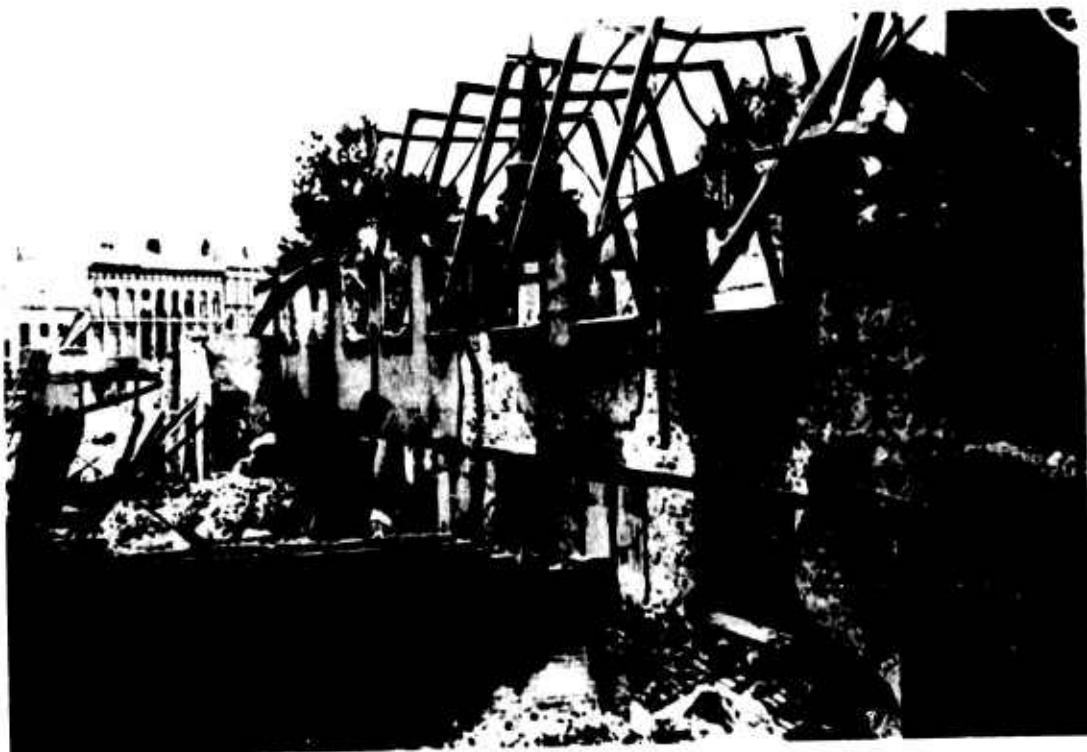
Picture 76 FIRE-DESTROYED ROOF OF NIGHTCLUB IN COOLSINGEL DISTRICT
