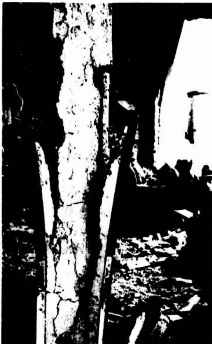
Picture 77 FIRE-DAMAGED CONCRETE PILLAR WITH BENT ANGLE-IRONS
