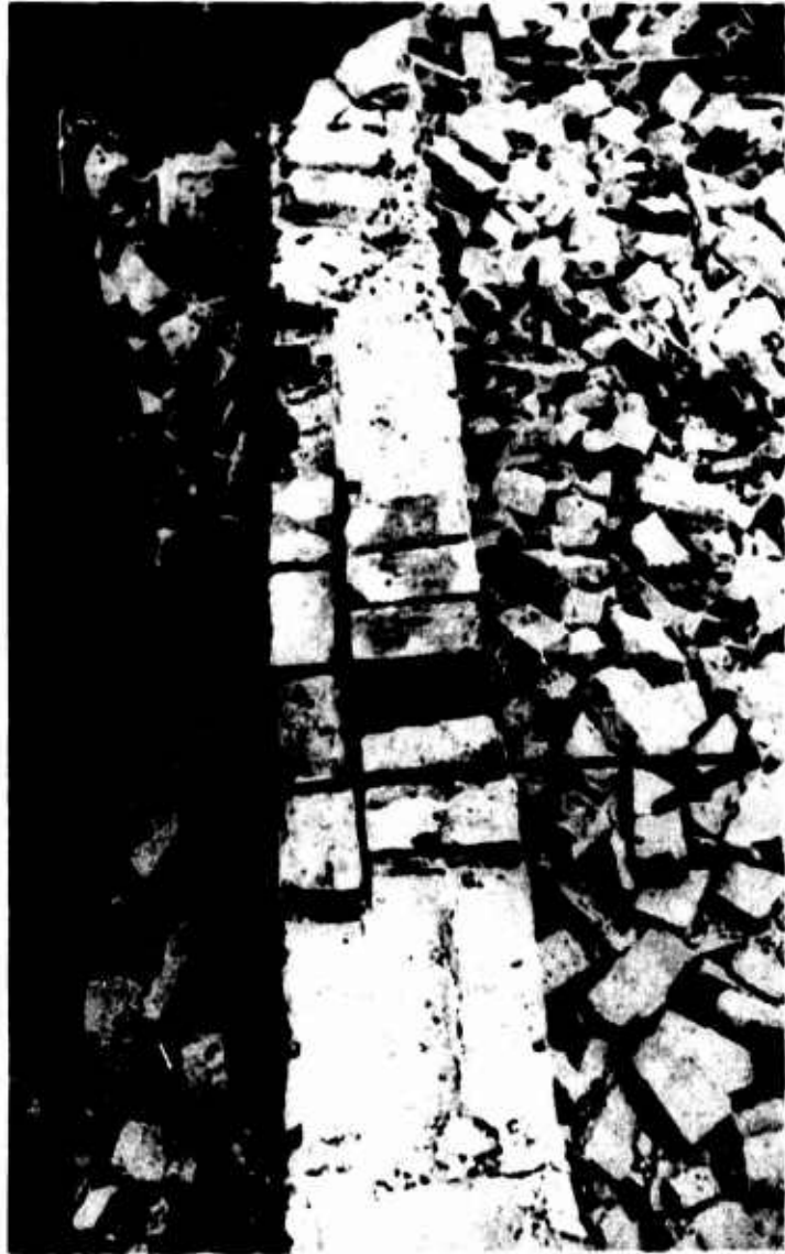
Picture 73 FIRE-DAMAGED BRICK FIRE WALLS (Note contiguous mortar layer between inner and outer wall)
