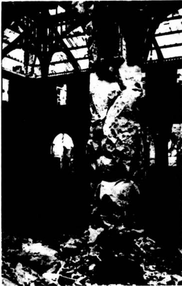
Picture 68 DAMAGED SANDSTONE COLUMN IN FIRE-GUTTED OLD STOCK-EXCHANGE BUILDING
