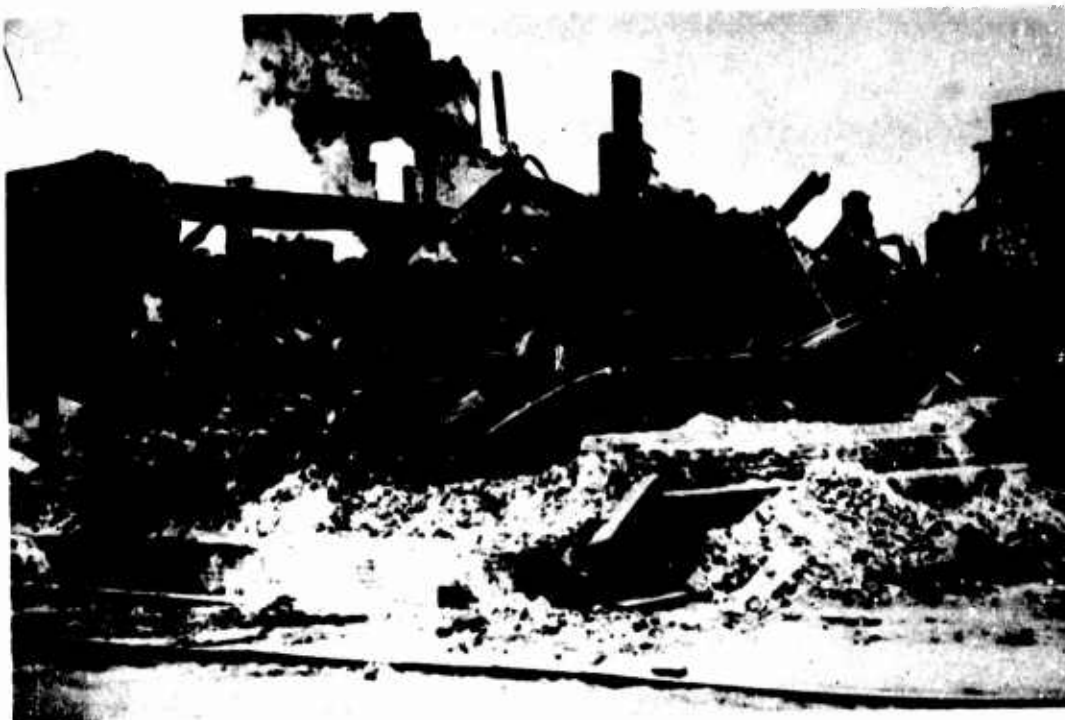
Pictures 35, 36 TWISTED STRUCTURAL STEEL, CHARACTERISTIC OF STRUCTURES DESTROYED BY FIRE
