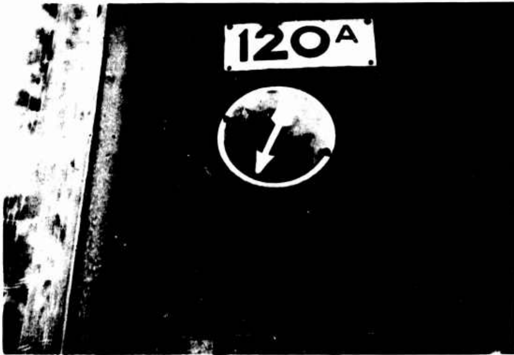
Picture 16 IDENTIFICATION OF UNDERGROUND FIRE HYDRANTS
