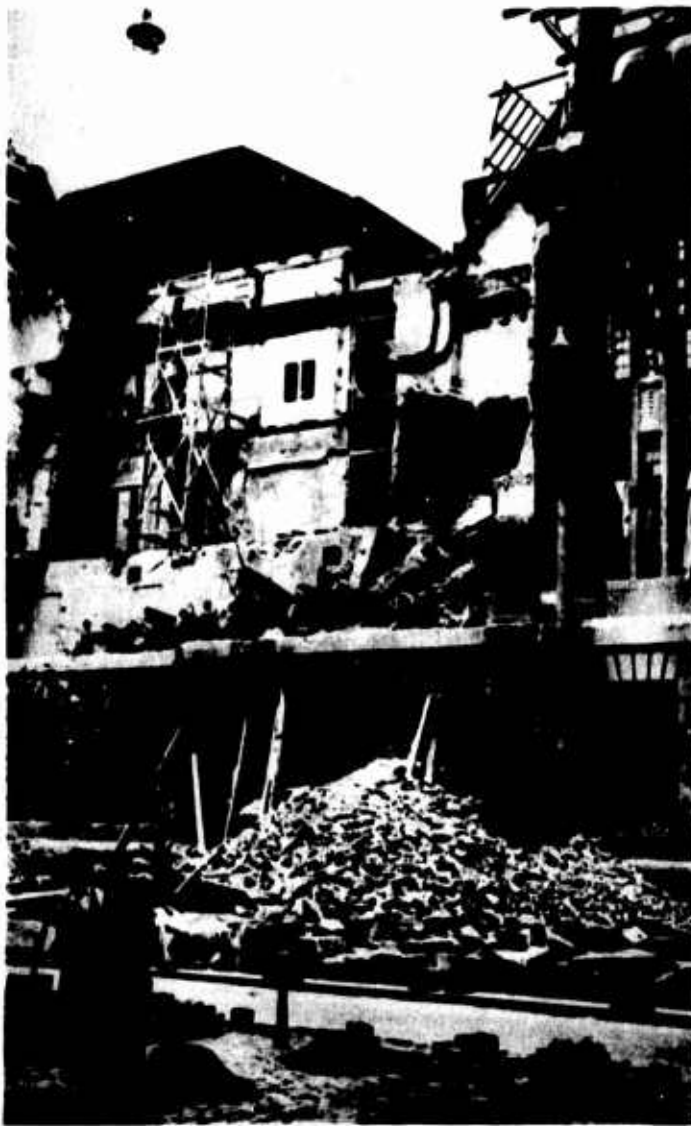
Picture 25 DIRECT HIT ON POST OFFICE BUILDING (NEXT TO THE CITY HALL; SEE CITY MAP, FIGURE 1). An example of pure high explosive bomb effects, i.e., hits from high explosive bombs that did not ignite.
