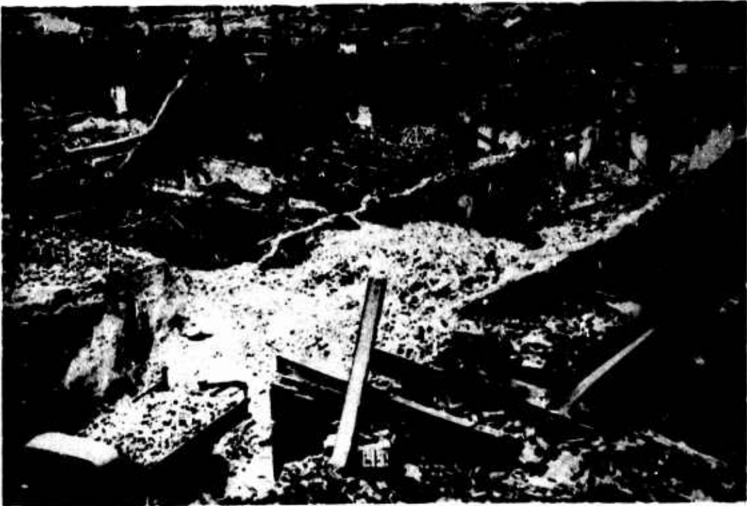
Pictures 31, 32 FIRE-DESTROYED STRUCTURES. All wooden parts, like beams, floors, doors, window frames, and shafts are completely burned. The fire sites are completely free of wood.
