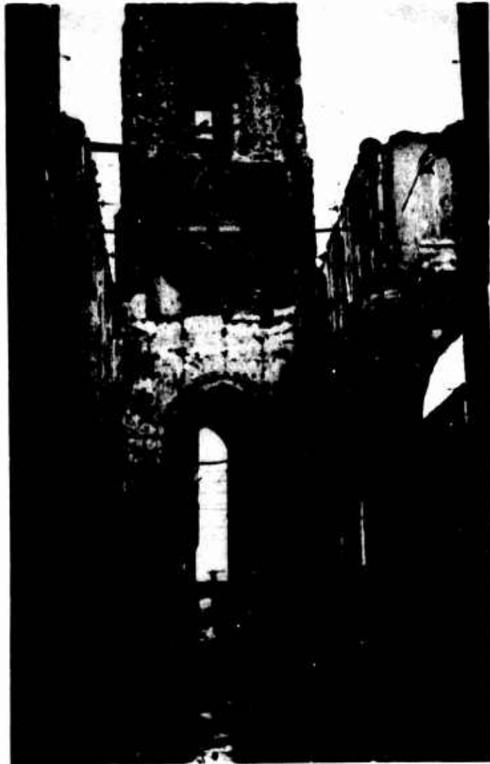
Picture 67 ST. LAURENS CHURCH SHOWING EVIDENCE OF FIRE-CAUSED SPLINTERING AND PEELING OF SANDSTONE
