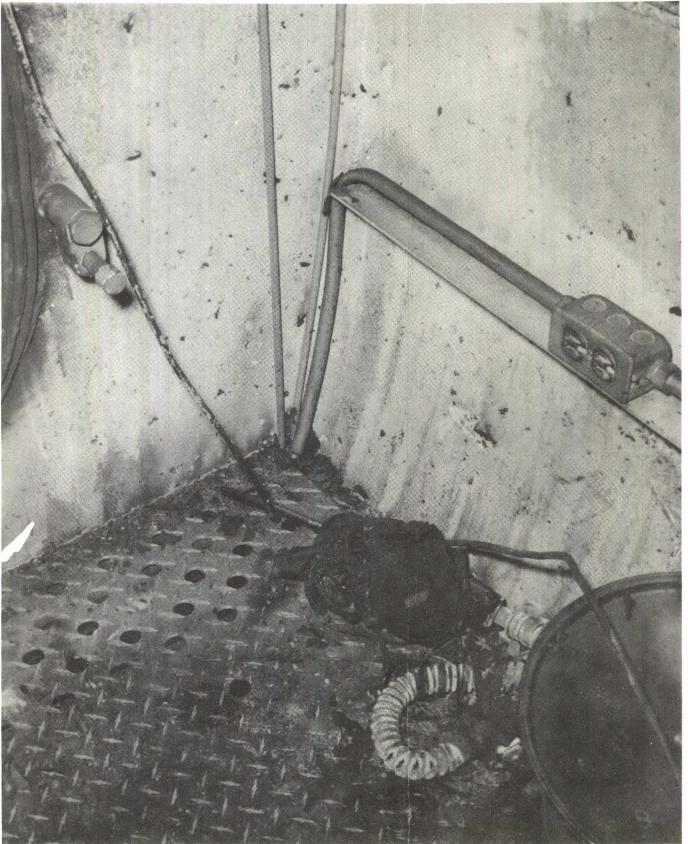
Figure 4 Right Rear Corner of Lock
